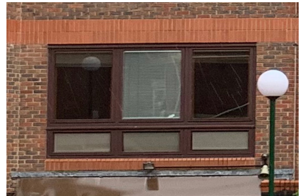
4. Existing ground floor window type
