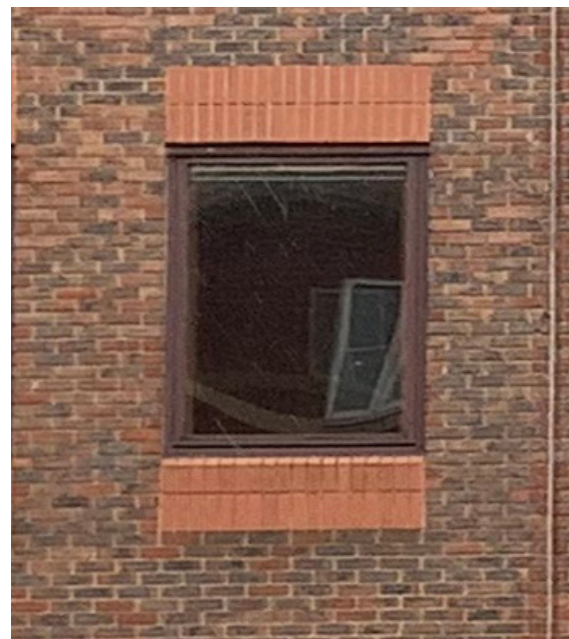
2. Existing window type
