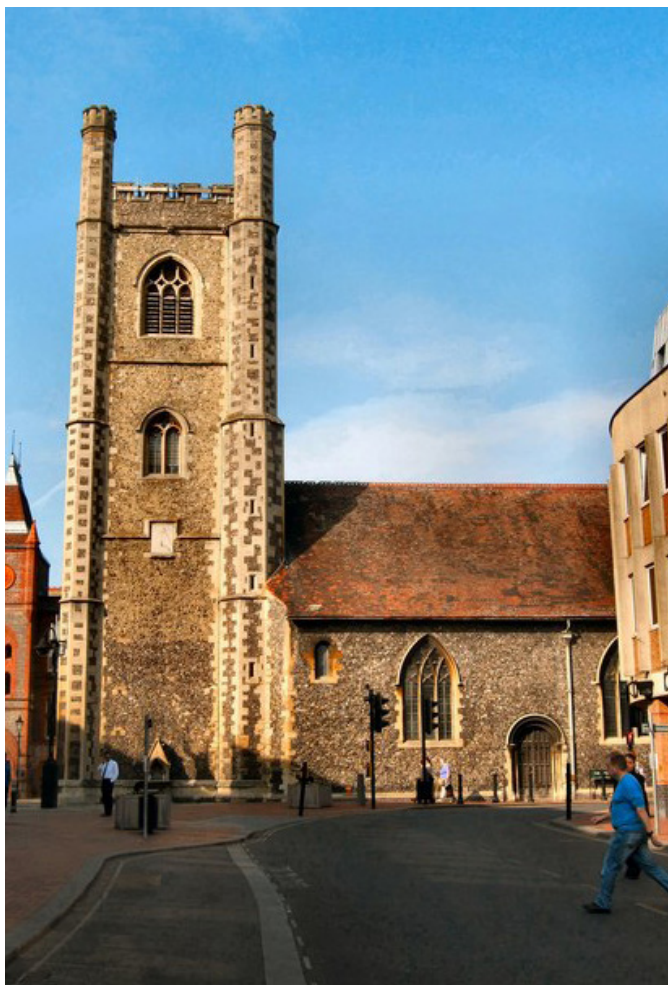
St Laurence's Church - Grade 1 listed building
