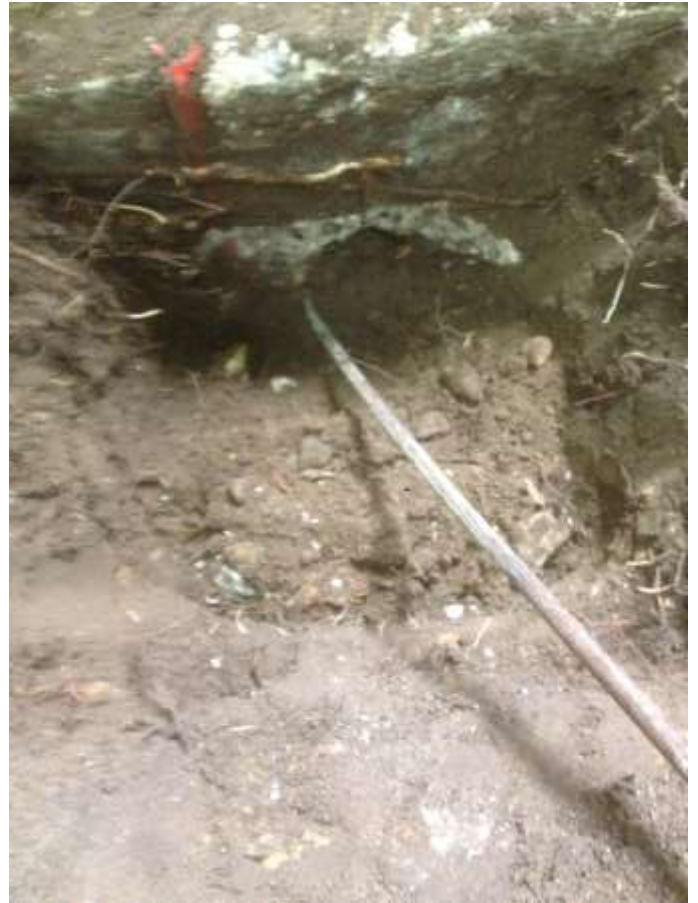
Photo 3 – EH2 Foundation Pit
