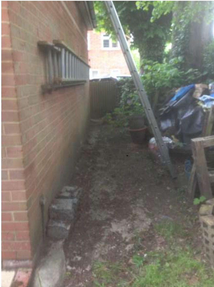
Photo 1 – Side elevation of garage
