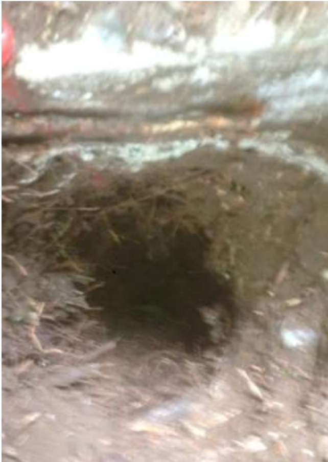
Photo 2 – EH1 Foundation Pit
