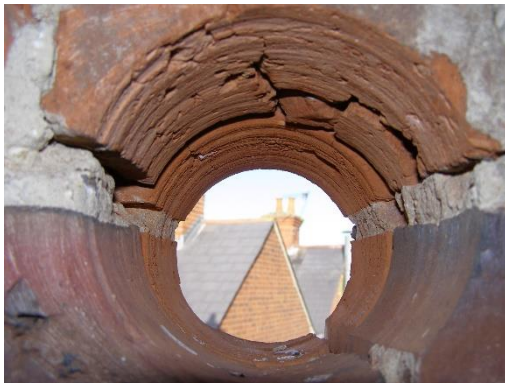
hole within no 1 loft space – direct access into loft space
