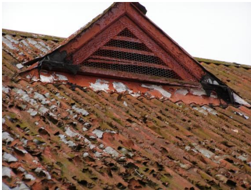
grated and wired vents of play barn roof
