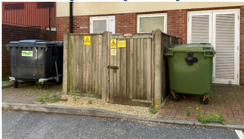
Figure 2 – Existing Refuse Storage
