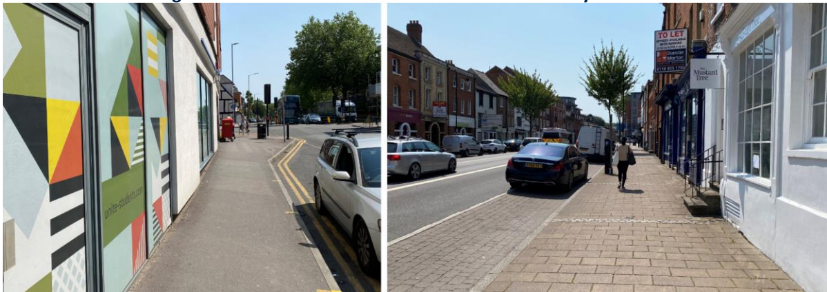
Figure 4 – Crown Street and London Street Footways
