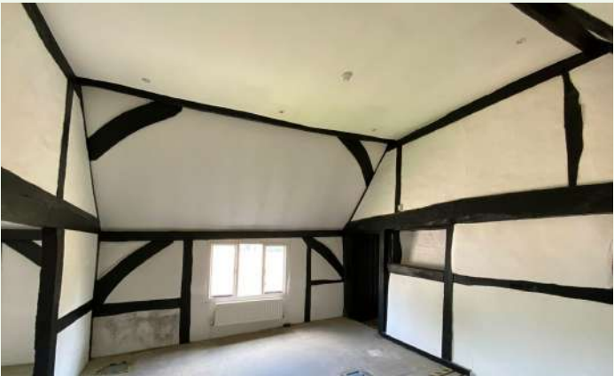
1/F INTERNAL VIEW
