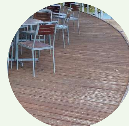
EXISTING TIMBER DECKING TO BE CLEANED AND RESTAINED
