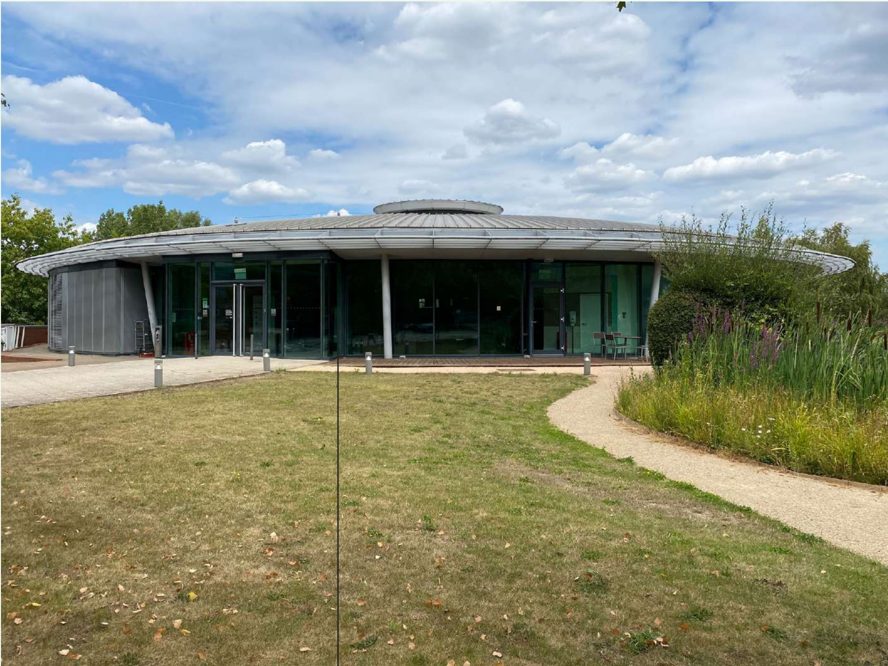
FRONT ENTRANCE ELEVATION
