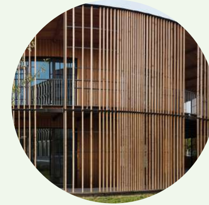
TIMBER CLADDING AS RAINSCREEN & ARCHITECTURAL SCREEN IN FRONT OF PLANT ROOM LOUVRES
