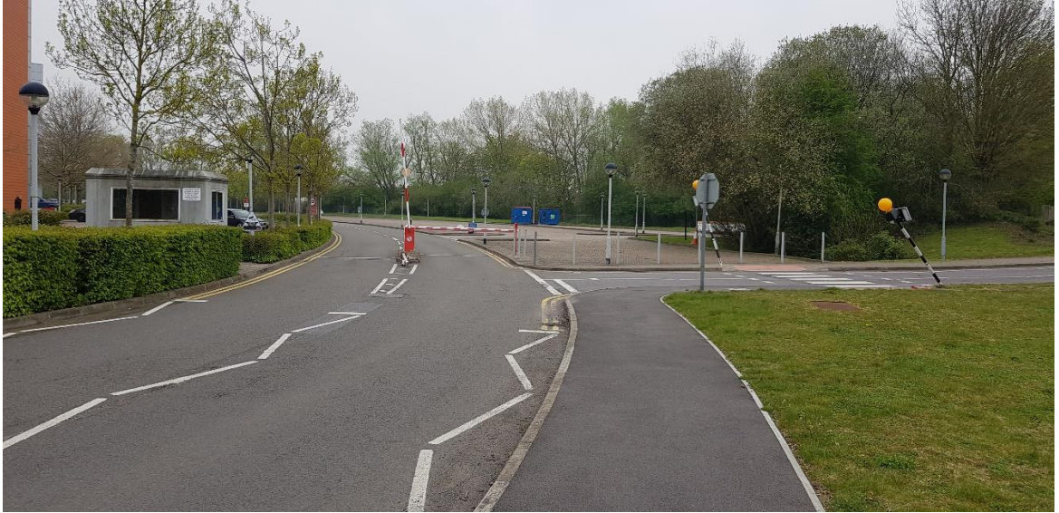
Figure 2-7: Damaged street furniture caused by manoeuvring lorries
