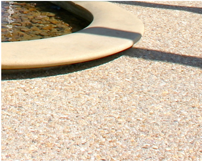
Fig. 3.6.3 - In Situ Concrete Finish
