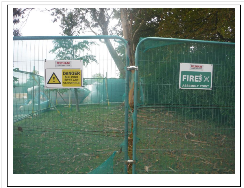
Heras with double clip system and bracing as per BS5837: 2012
