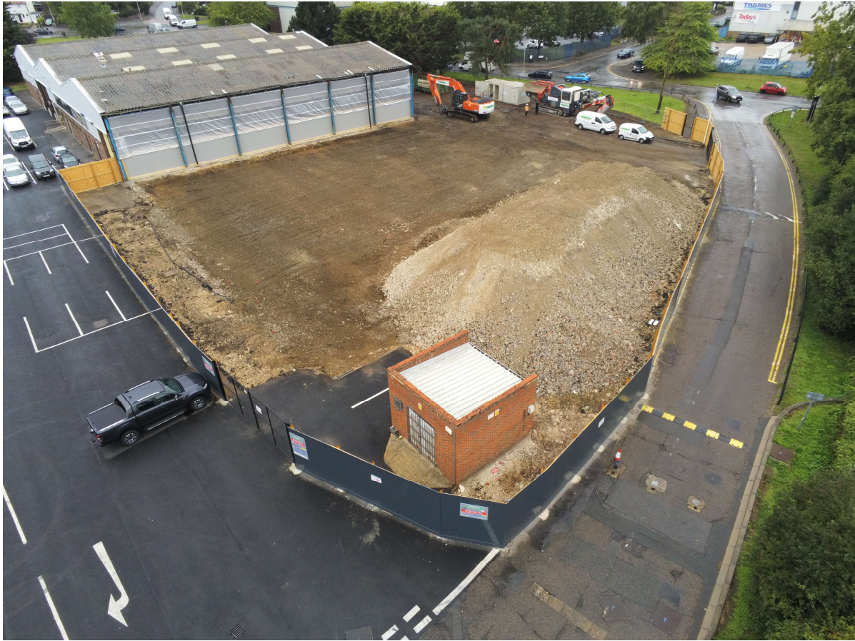
FIGURE 2: EXISTING SITE PHOTO (LOOKING SOUTHWARD)
