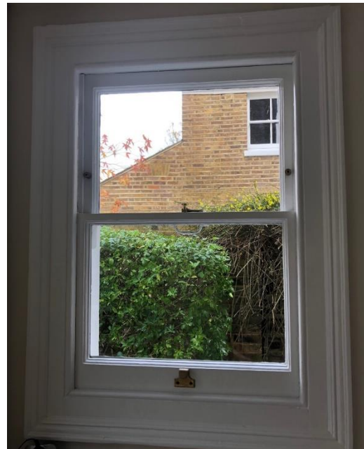
Two kitchen windows (larger and smaller) at the back of the property
