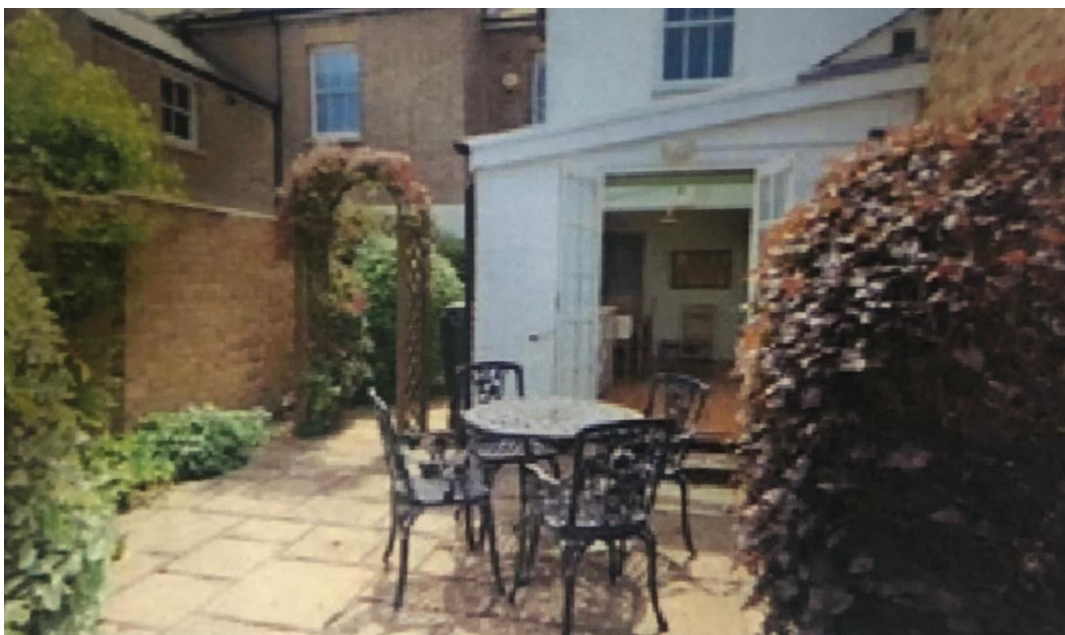
Rear of the property: Photo shows rear access and also 1 st floor bathroom window
