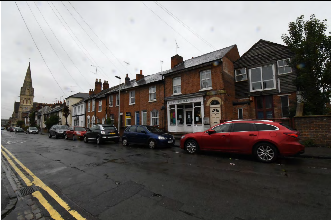
Plate 13 The Front Elevation of the terrace
