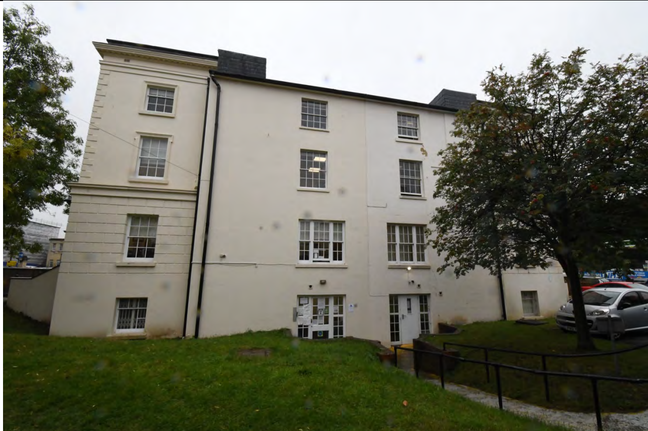
Plate 10 The Front Elevation of The Building
