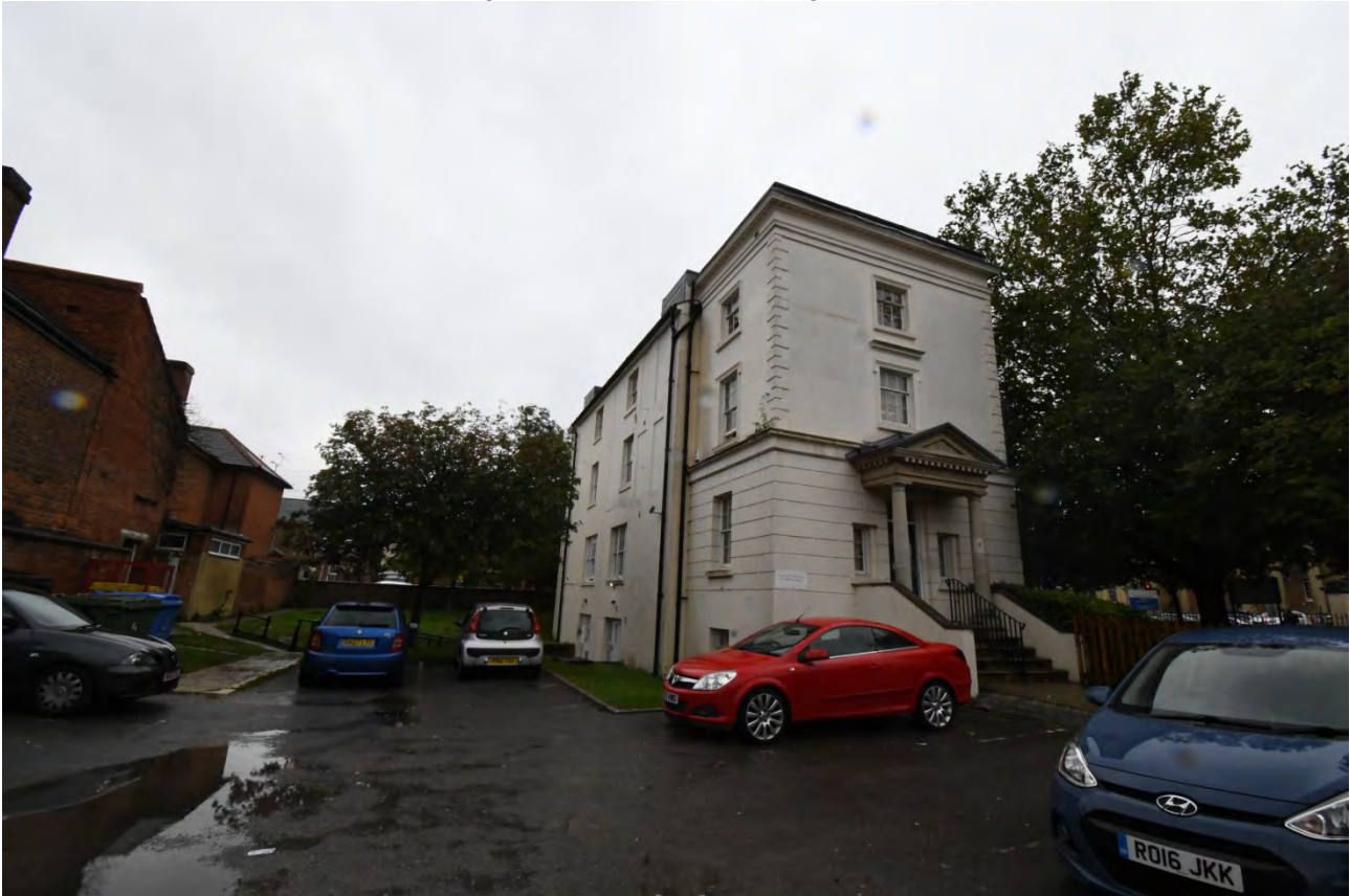
Plate 12: The west elevation of the building with the surrounding car park which replaces the formal gardens
