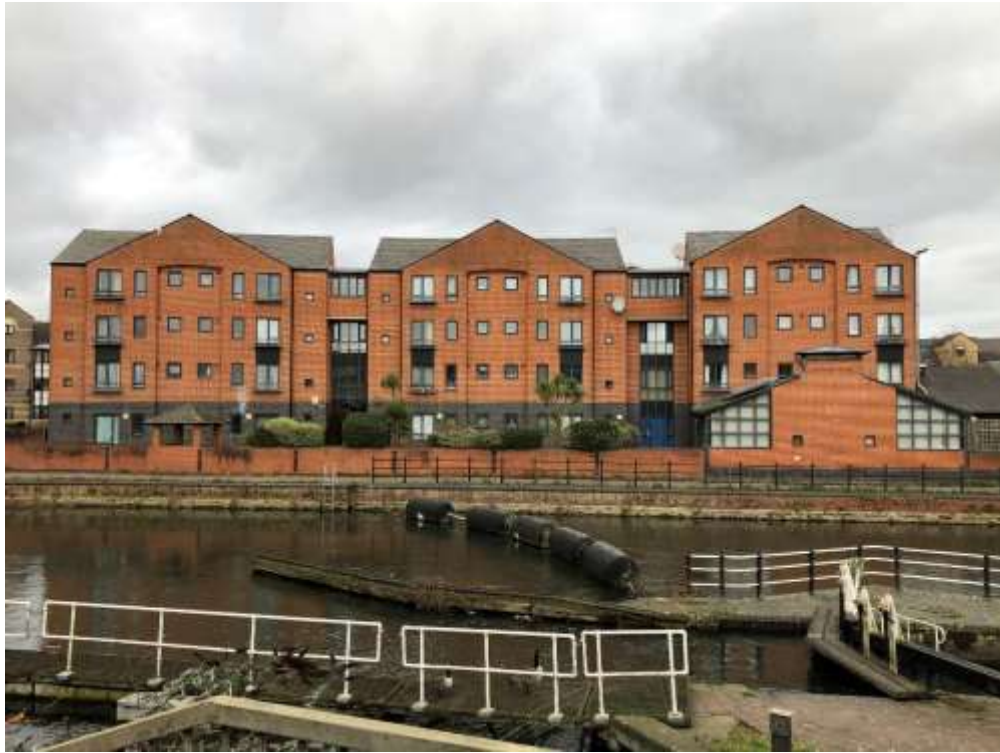
3. View of existing Rear Elevation (South-East facing).
