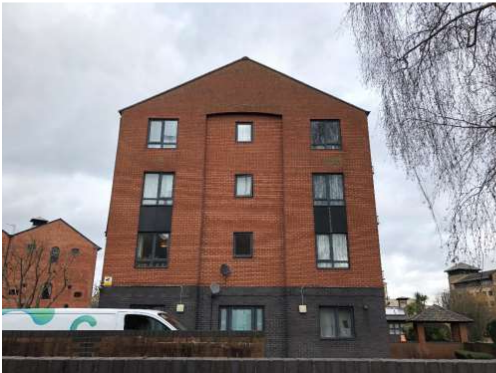
2. View of existing Side Elevation (South-West facing).
