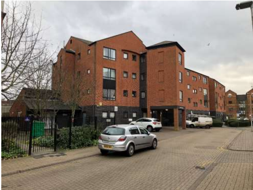
1. View of existing Front Elevation (North-West facing).
