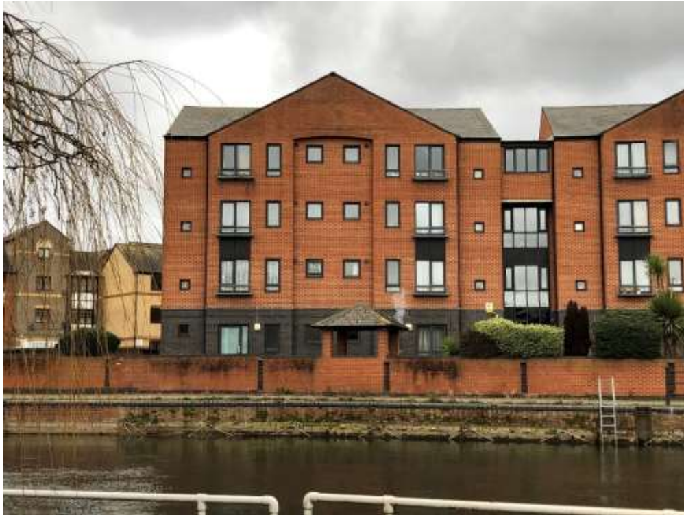
5. View of Rear Elevation of Wardens Flat (Ground Floor).
