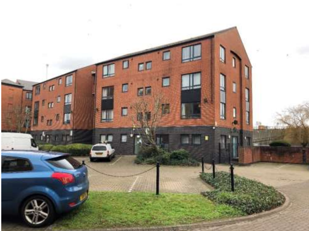
4. View of Front Elevation of Warden's Flat (Ground Floor).
