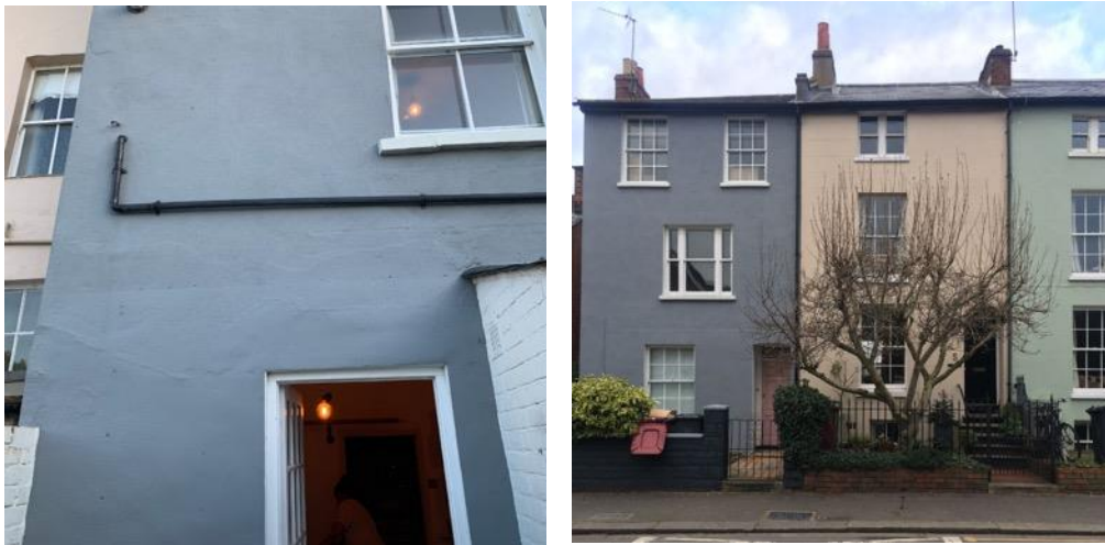
Figure 2 - Repainted stucco on the front and rear facade
