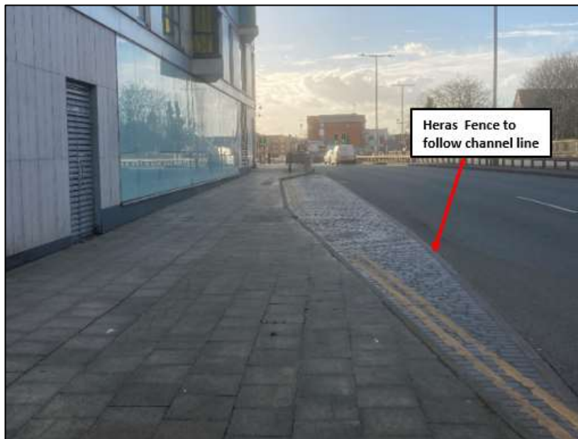
Figure 5.3 – Heras Fence Line, Chatham Street
