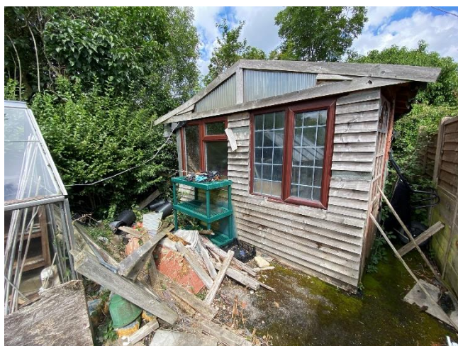
Photo 7: Wooden storage shed located in the northeast area of the survey site.
