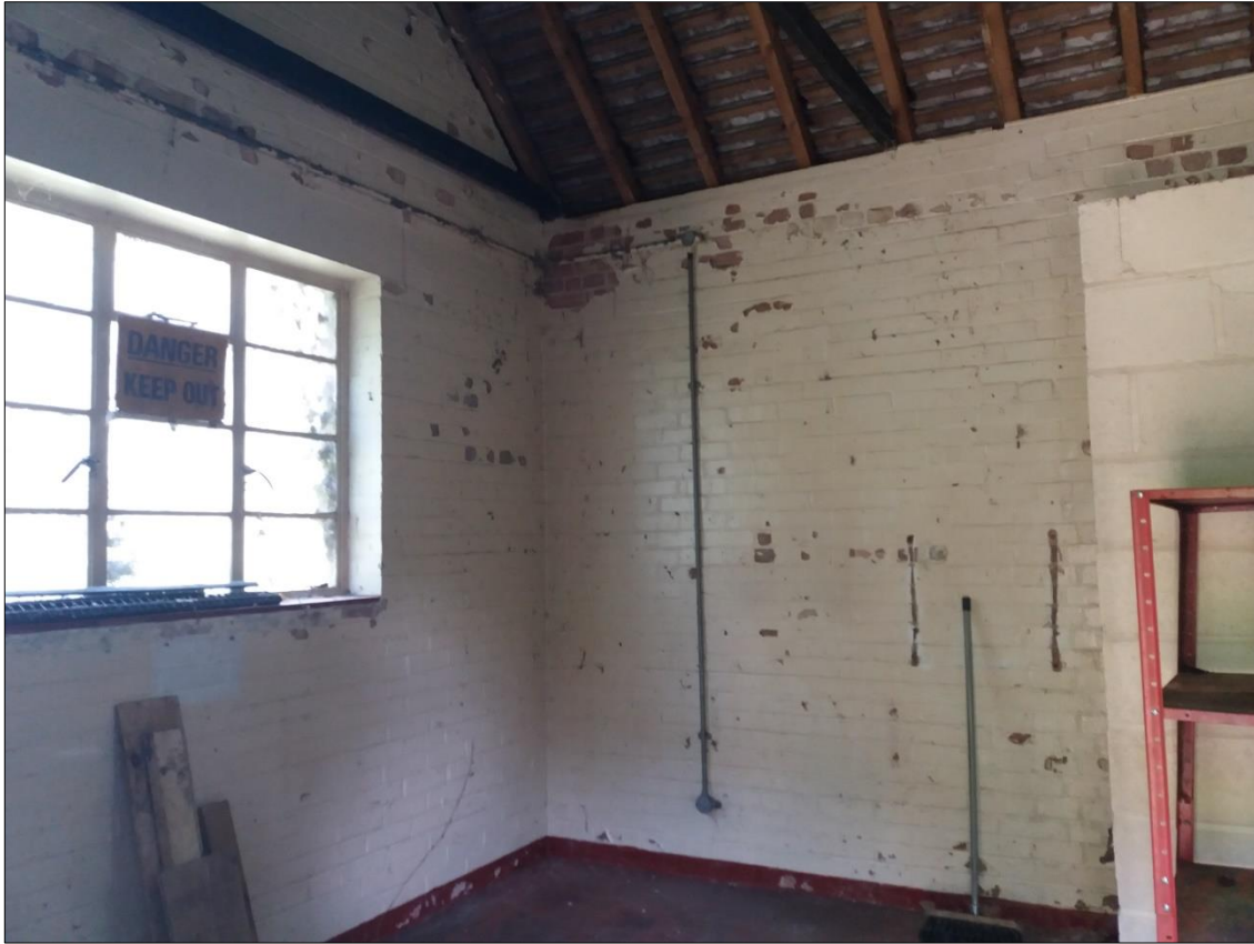
FIGURE 3A - INTERIOR VIEW SHOWING THE DISUSED BUILDING
