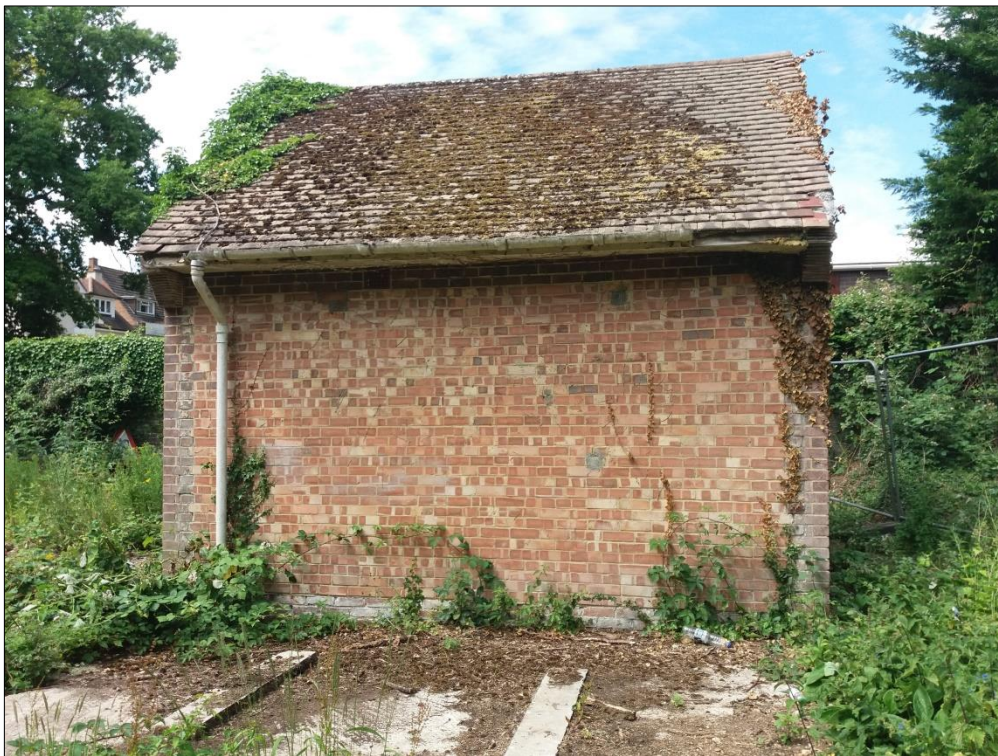
FIGURE 3 – EXTERNAL VIEW OF THE PUMPING STATION BUILDING
