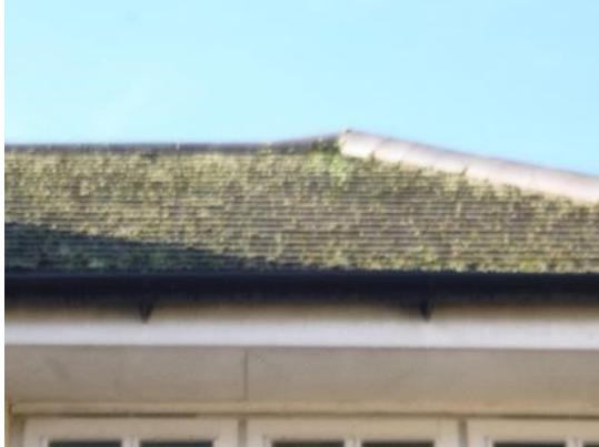
11. Tight roof tiles on the north-eastern side of the house: soffit flush with the wall.
