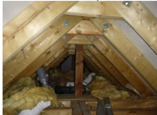
16. Hipped roof extensions with intact breathable membrane lining.
