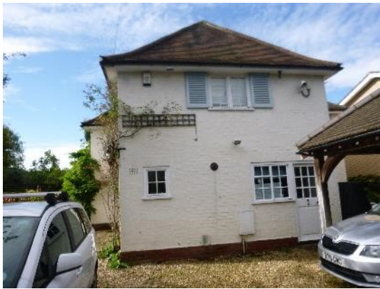
1. Front of the house viewed from the northeast.
