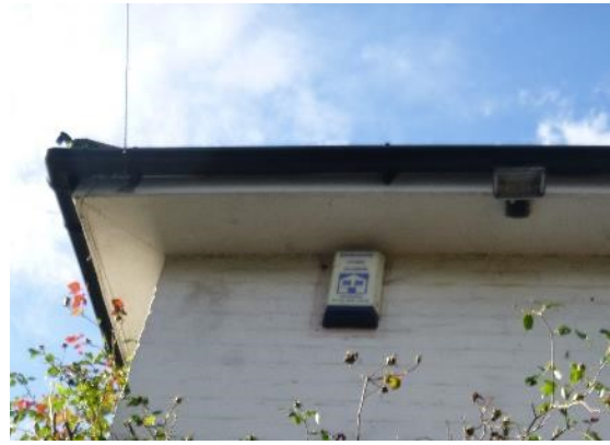
4. Tight wooden soffit, flush to wall.
