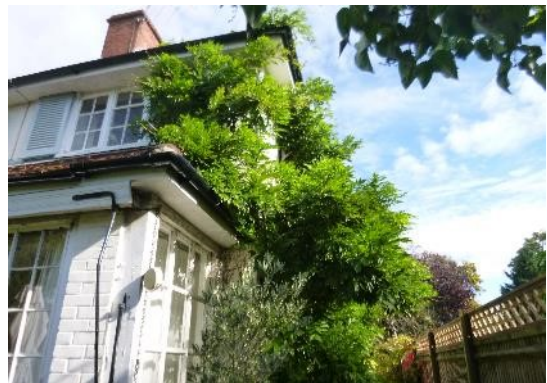
6. Tight lead flashing around base of chimney; slightly lifted tile below chimney.
