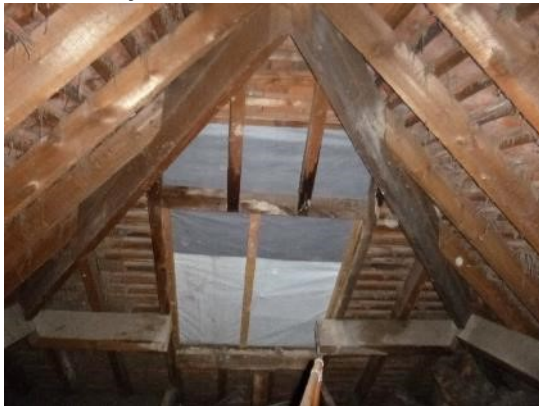
19. Area of hipped roof covered in plastic sheeting and breathable roofing membrane.
