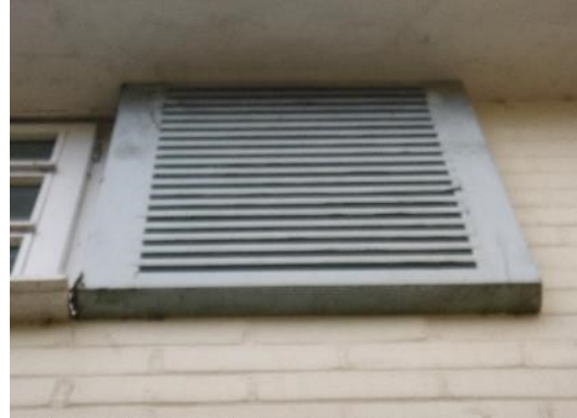
12. Open shutters on windows, with no promise for roosting opportunities.
