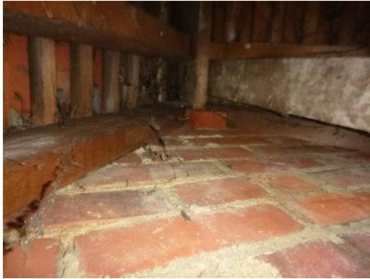
17. Beams and rafters tight to brickwork around the chimney.
