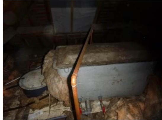
18. Covered water tank to the north-eastern end of the void.
