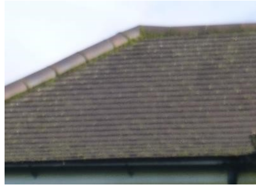
10. Flat and intact roof, verge and hip tiles on the newer extension to the northern side of the house.
