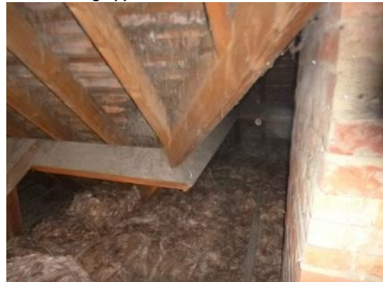
14. Newer fibreglass insulation laid to the south of the void around the chimney.
