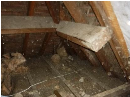
15. Older fibreglass insulation around the loft hatch and to the north-eastern side of the void.
