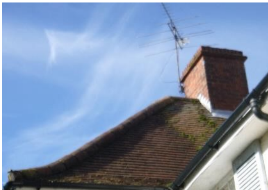
5. Tight lead flashing around base of the chimney; Intact hip, ridge and flat roof tiles.
