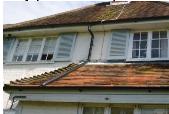
8. Tight wooden soffit around the rear elevation of the house.
