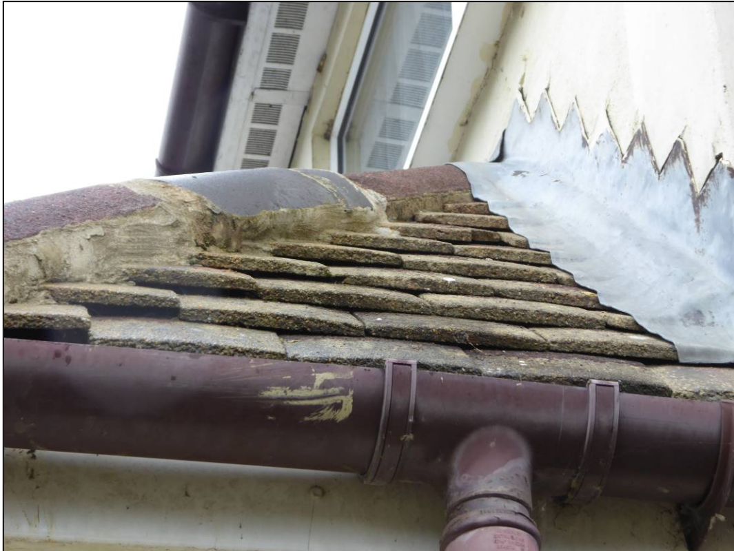
Figure 14. Example of lead flashing, 36A Mill Road, Caversham. 19.08.20
