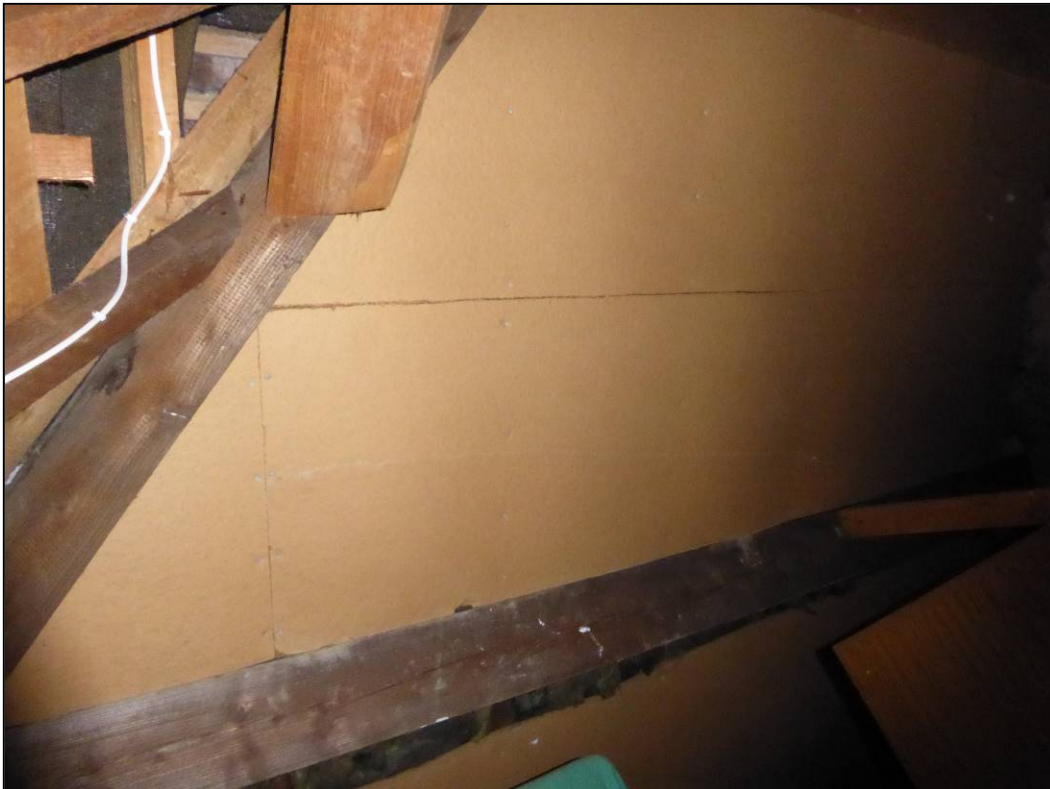
Figure 20. Example of wooden boarding. 36 Mill Road, Caversham. 19.08.20
