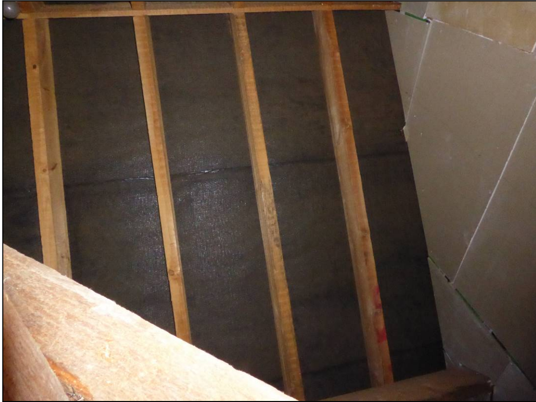
Figure 21. Example of bitumen lining, 36 Mill Road, Caversham. 19.08.20
