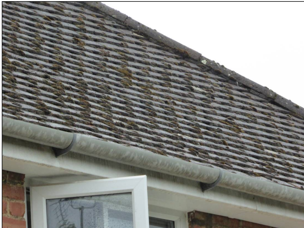
Figure 11. Example of roof tiles, 36 Mill Road, Caversham. 19.08.20
