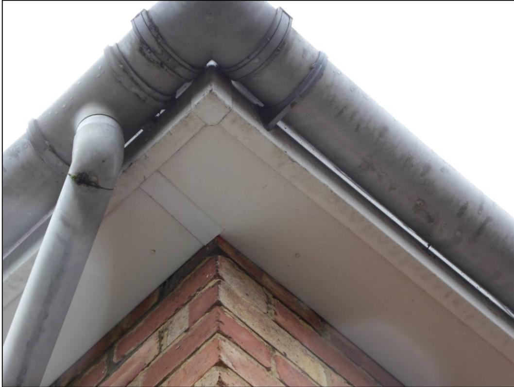
Figure 8. Example of fascias and soffits. 34 Mill Road, Caversham. 19.08.20
