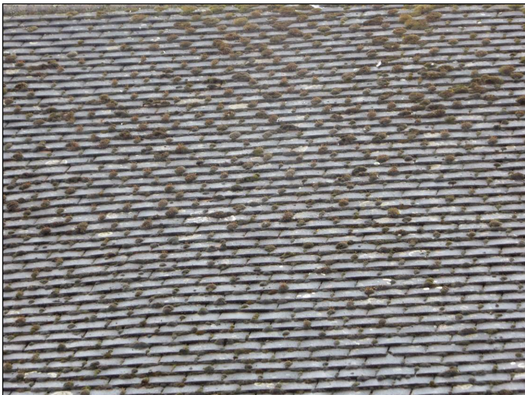
Figure 7. Example of roof tiles. 34 Mill Road, Caversham. 19.08.20
