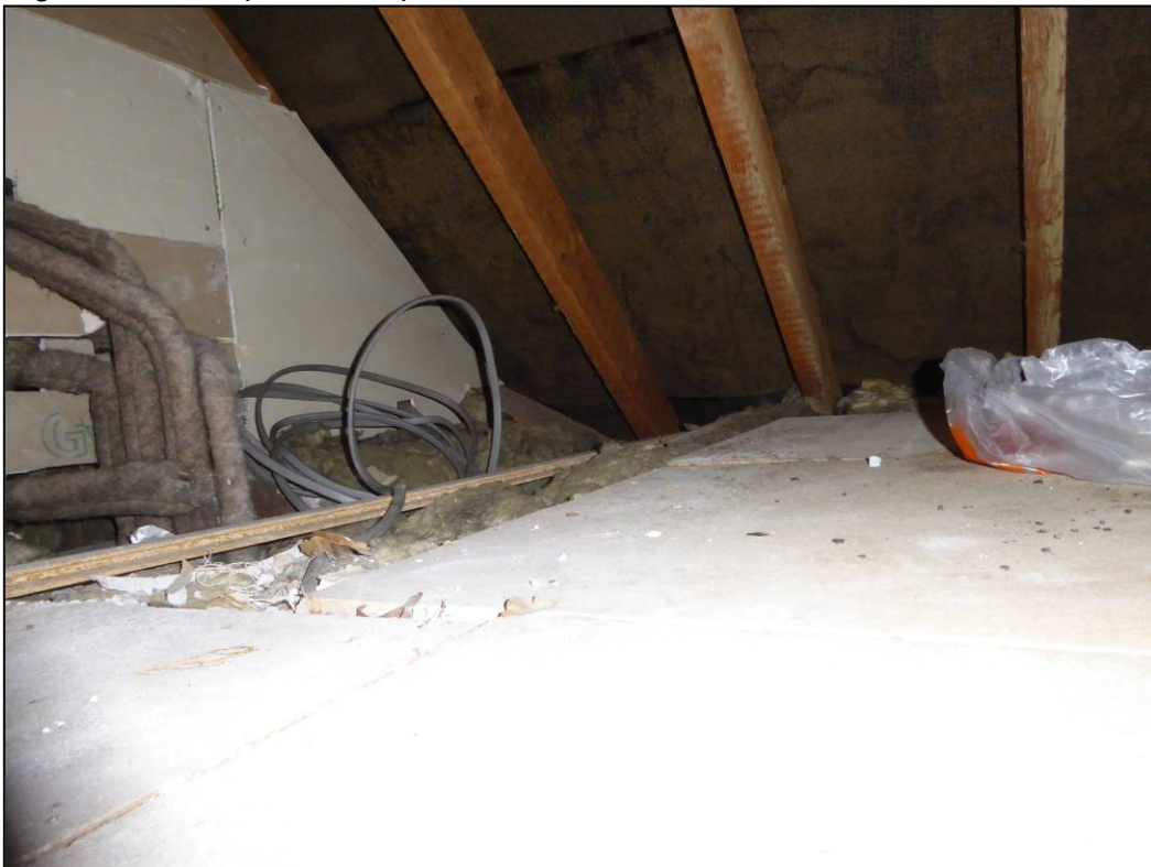
Figure 22. Example of loft space. 36A Mill Road, Caversham. 19.08.20
