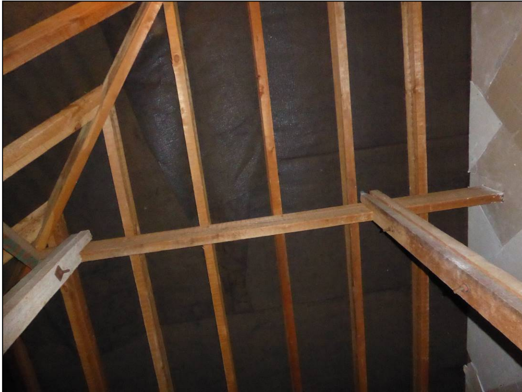
Figure 23. Example of bitumen lining. 36A Mill Road, Caversham. 19.08.20
