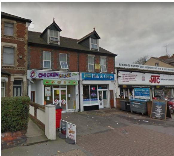
Figure 1 – Street view of 263 and 265 Oxford Road. 265 Oxford Road is on the right hand side
