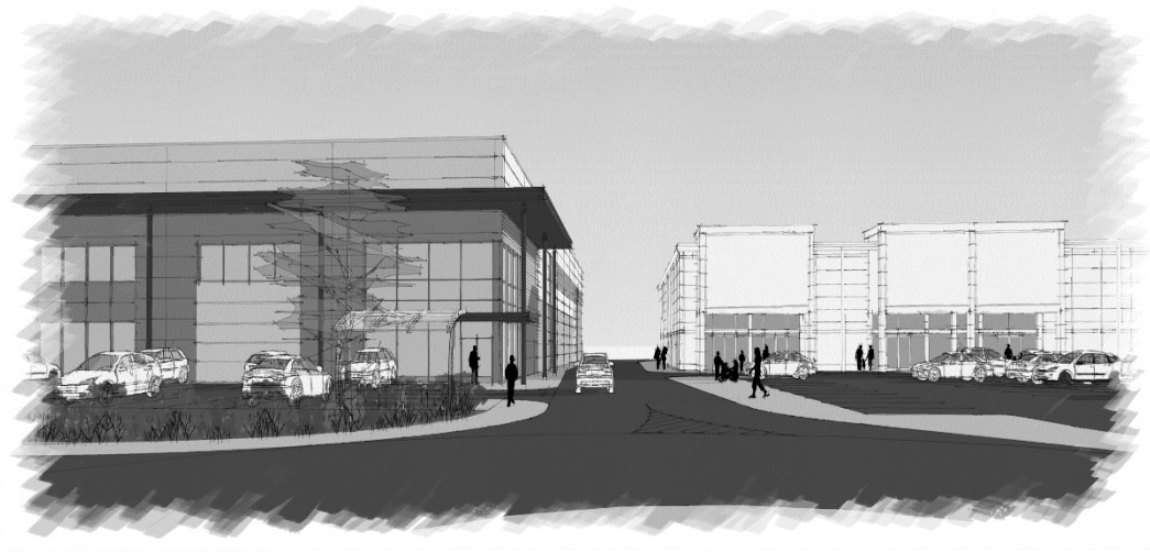
Fig. 6 View South East from Retail Park Entrance
