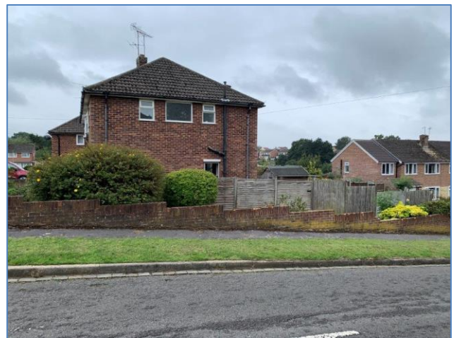
2. Front and side of 36 Elmstone Drive. Photo provided by the agent on 13/11/2020.
