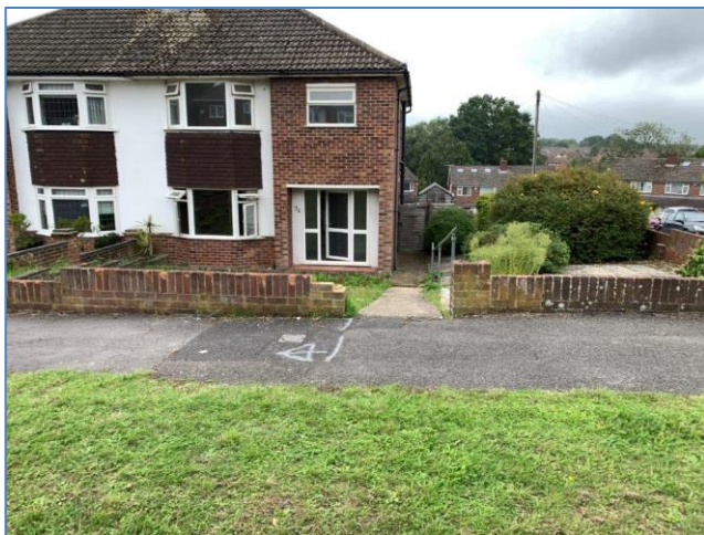
1. Front of 36 Elmstone Drive. Photo provided by the agent on 13/11/2020.
