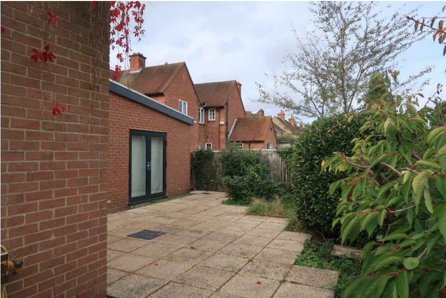
Looking along rear elevation
