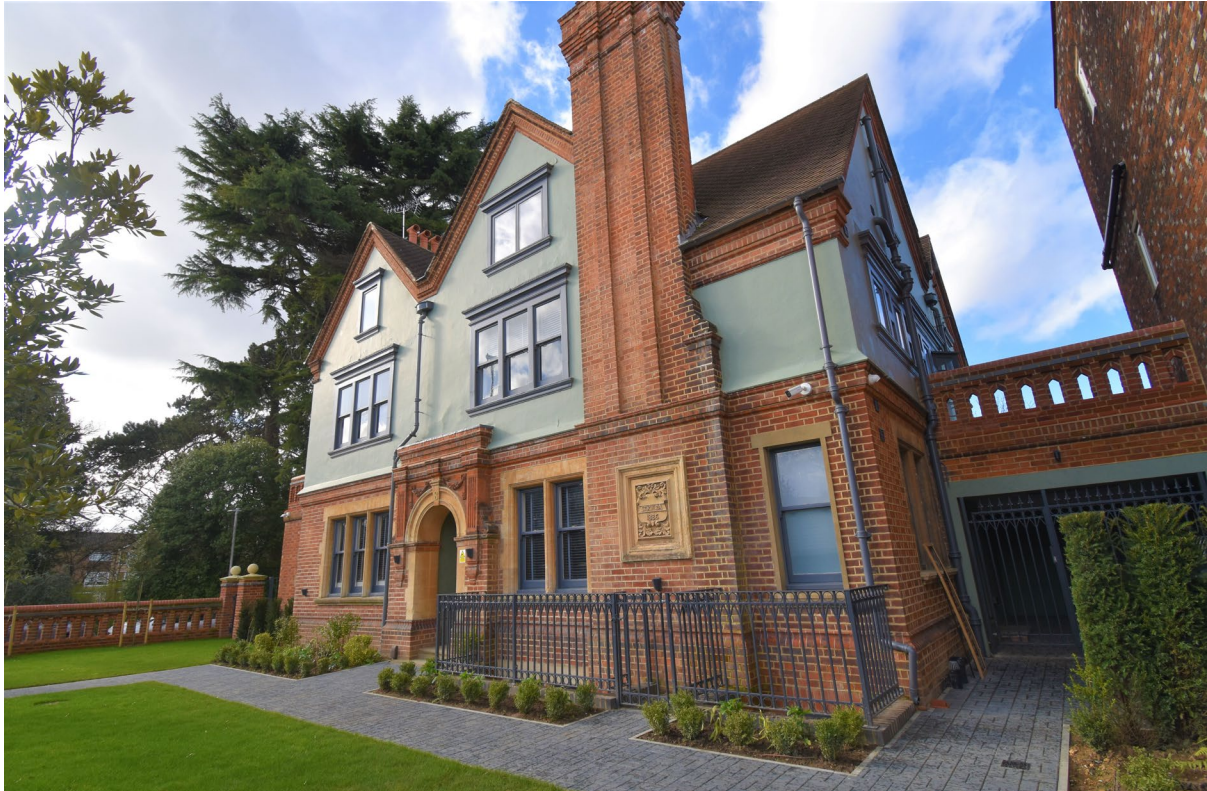
Exterior View of HMO at 8 Bath Road, Reading.
