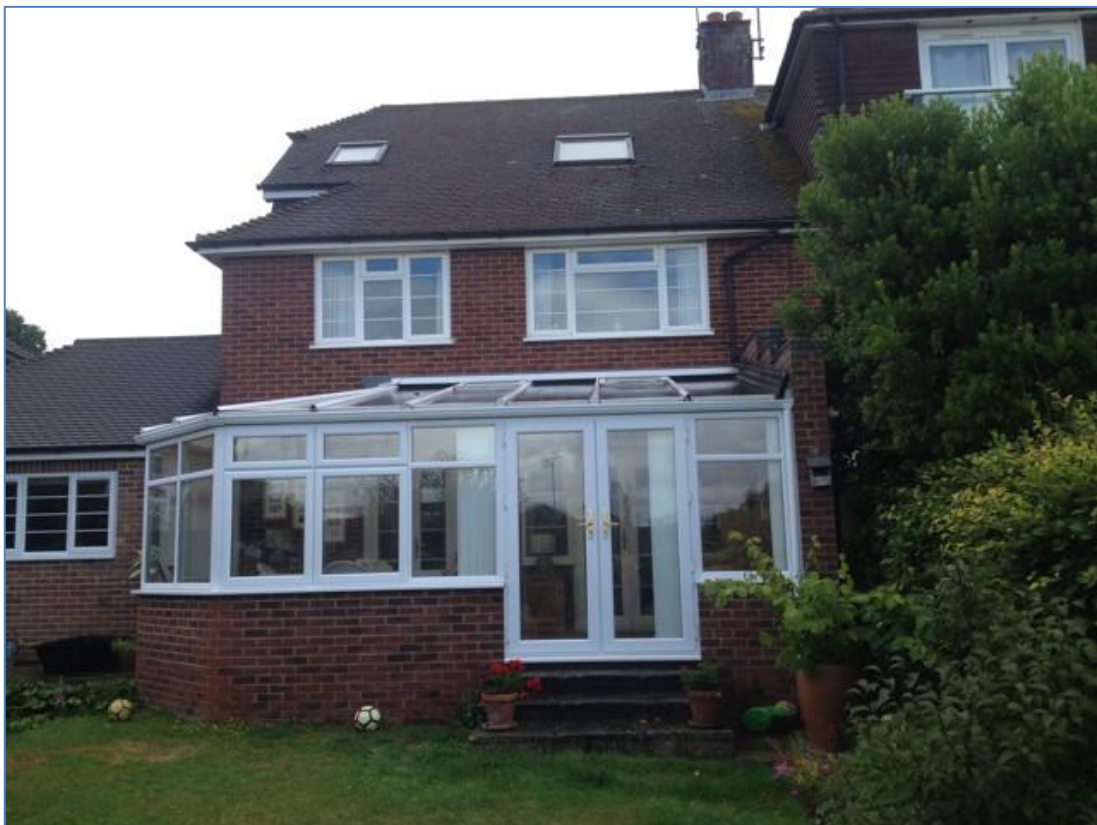
1. Existing conservatory at 11 Crawshay Drive, adjoining property is 9
