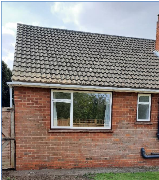
Fig 1. Rear of 107a St Michaels Road. Site photo provided by agent on 16/11/2020.
