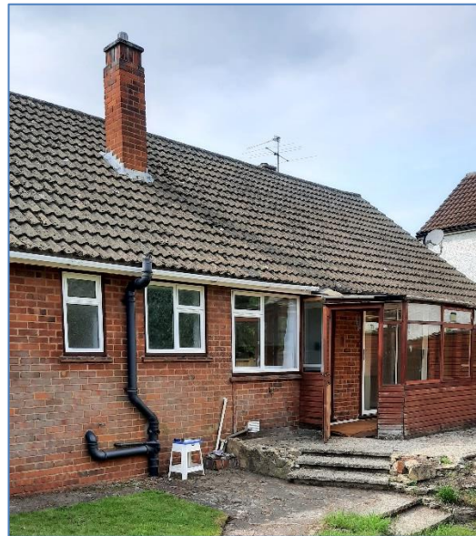
Fig 2. Rear of 107a St Michaels Road. Site photo provided by agent on 16/11/2020.
