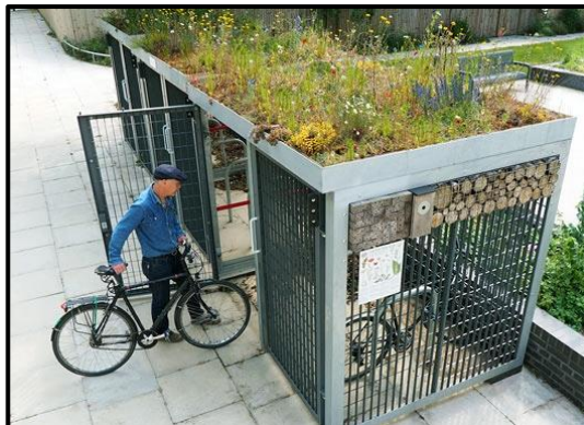
Photo 5.2: Cycle store with a green roof, invertebrate houses and bird boxes installed within the walls (Green Roof Shelters, 2016).
