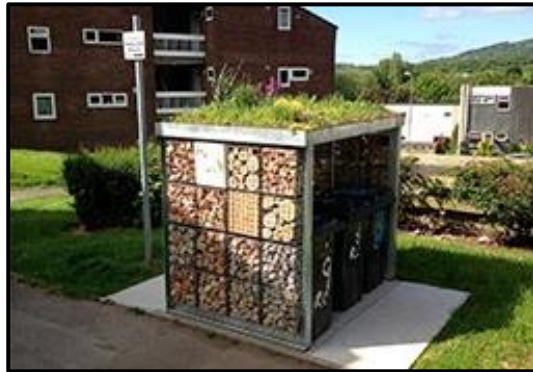
Photo 5.1: Bin store with a green roof and invertebrate houses in the walls (Green Roof Shelters, 2016).
