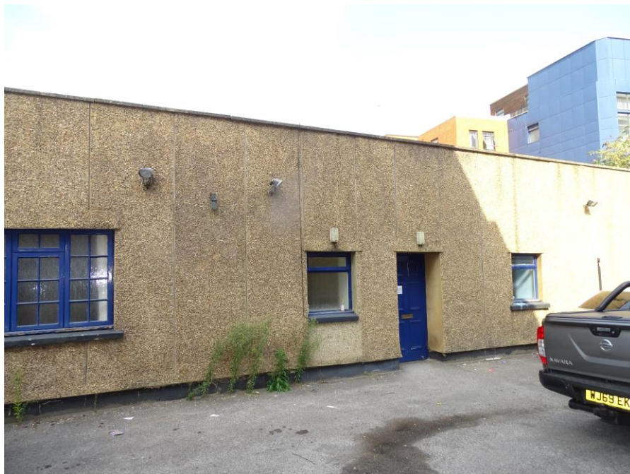
Photo 1: Building 1, southern elevation facing north.
