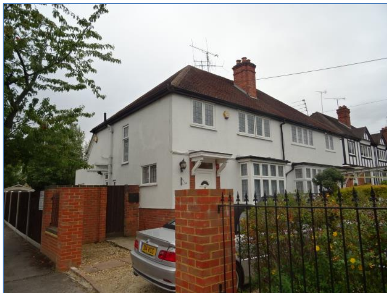
Fig 1. Front of 220 Norcot Road. Site photo provided by agent on 08/12/2020.
