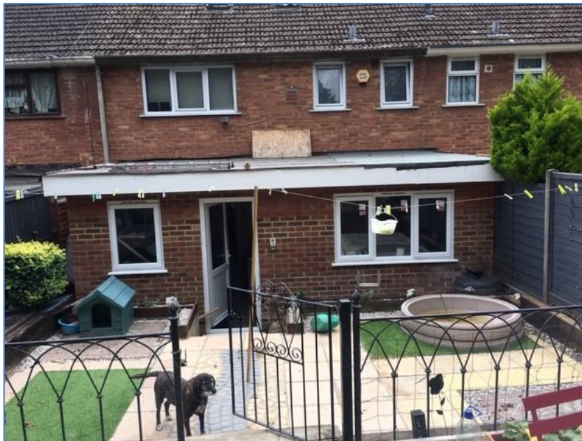
Rear of 214 Wensley Road. Photo provided by the applicant on 16/07/2020. Existing ground floor rear extension approved under planning application 171036 on 26/07/2017 (see 'Relevant Planning History' for details).
