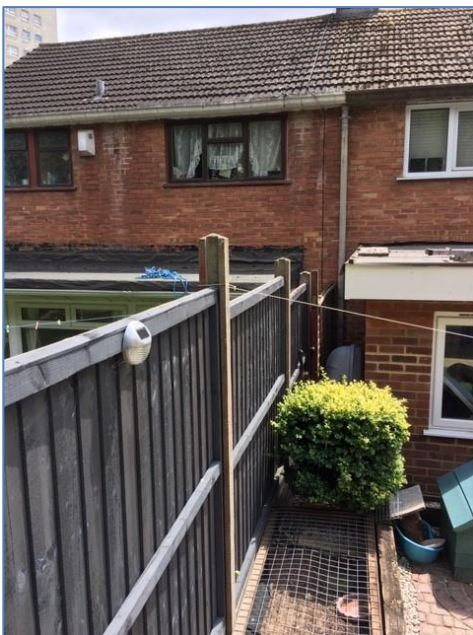
Fig. 2 - Rear elevation of 212/214
