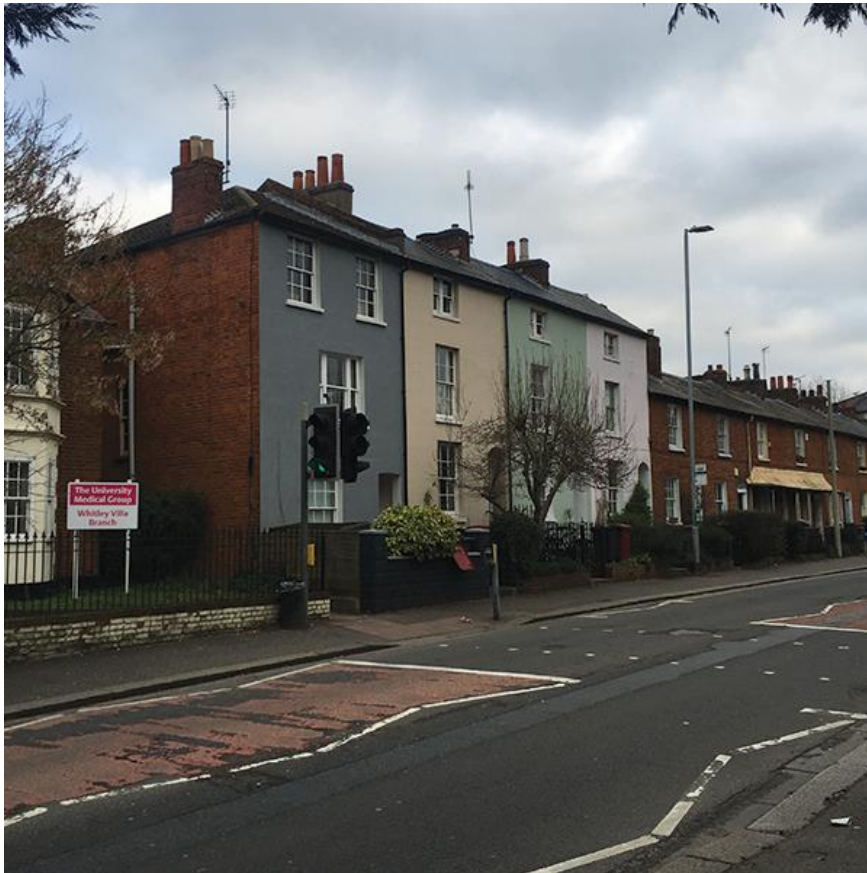
Figure 1 - Street view of No.3 along Christchurch Road (painted in mid-lead)
