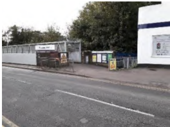
Tilehurst Road/platform 1 access
