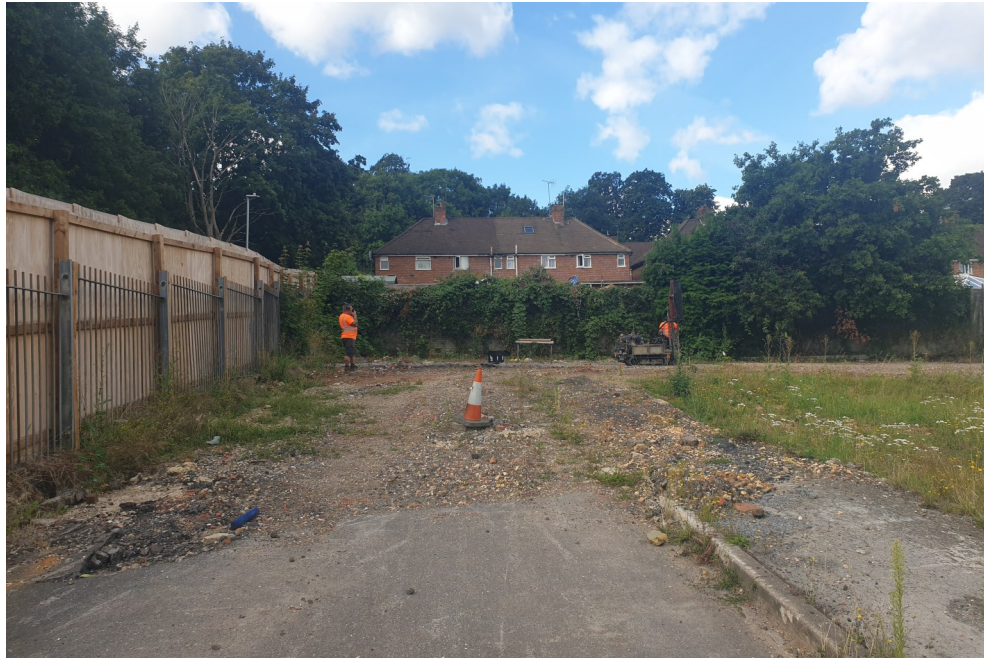
View looking southwest from gate within hording.
