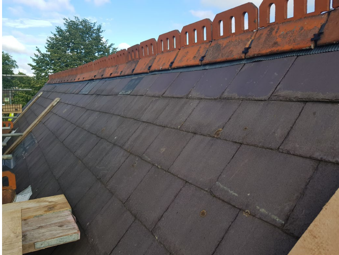
Fig 3: Roofing slate to match existing
