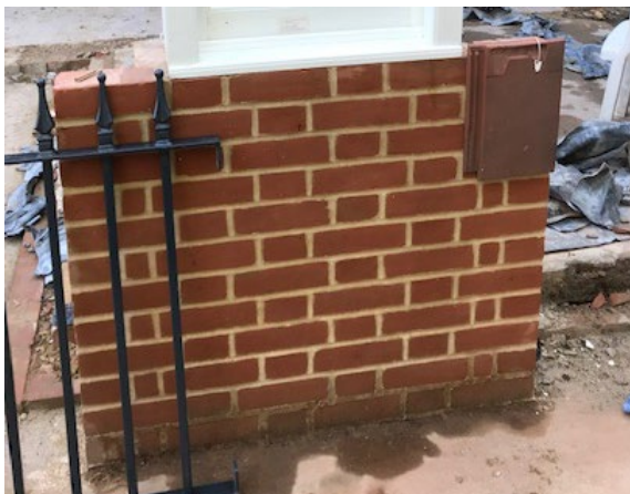
Fig 1: Brick sample panel
