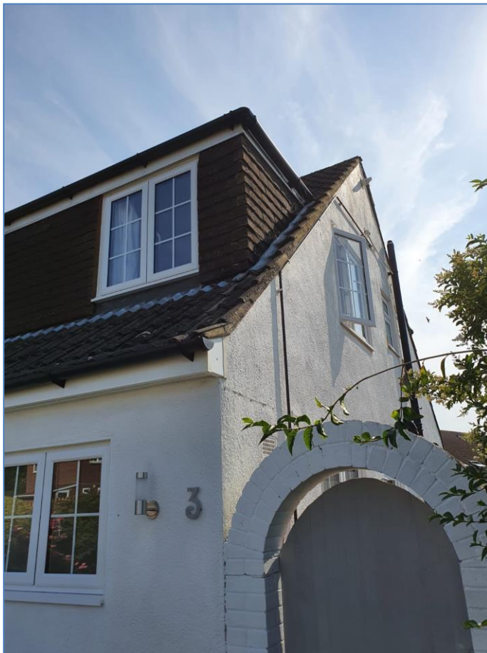
1. Front/side elevation of 3 Alandale Close (photo provided by agent)
