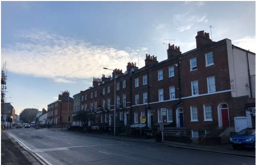
Figure 11: View of Grade II* 78 – 84 Southampton Street
