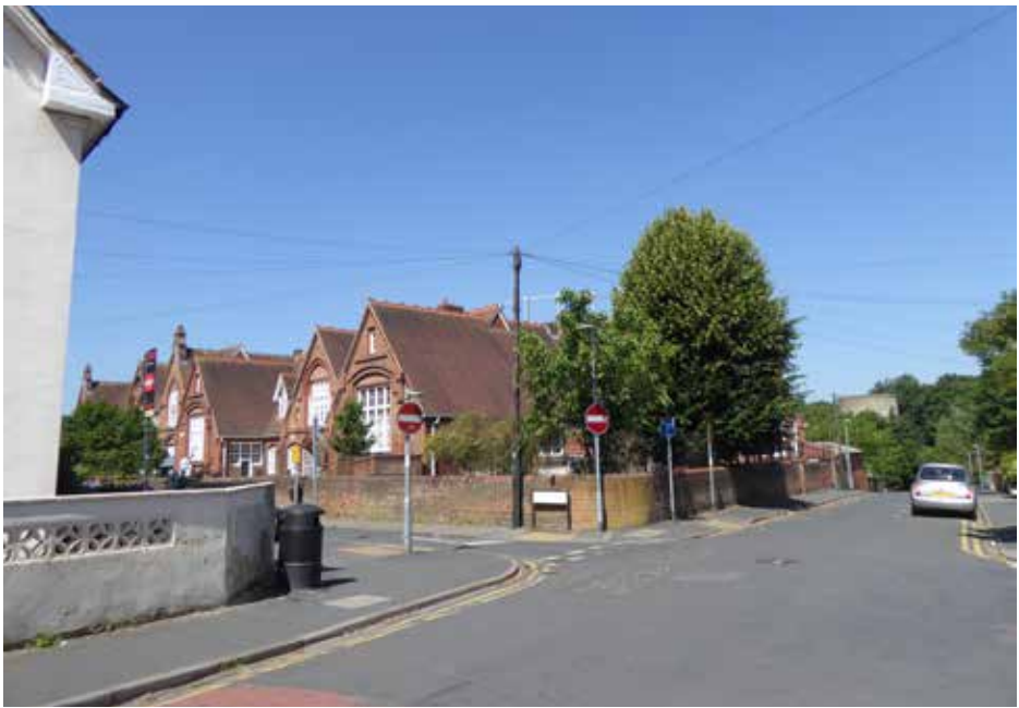
Figure 5.6 The view of Newton School (Grade II) from the south east. The gas holder is glimpsed in this location and is clearly identifiable as an industrial feature that contrasts with and is later than the school.
