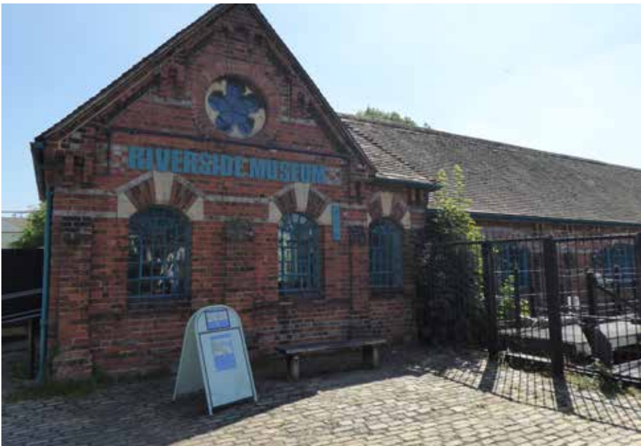
Figure 5.8 The north end of the Pump House and Turbine House (Grade II).
