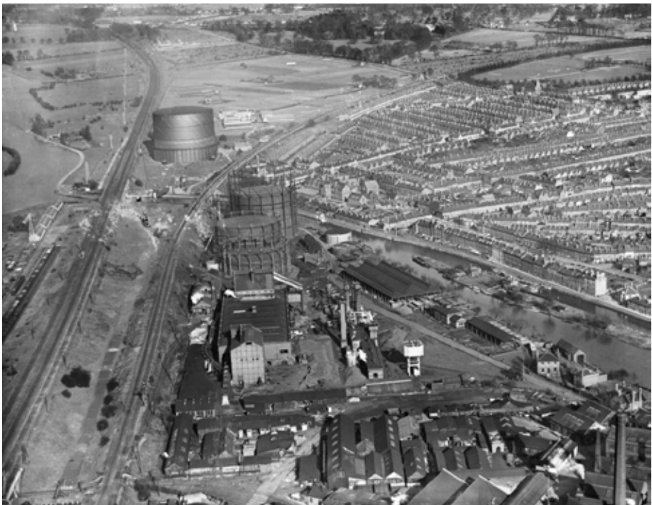
Figure 4.6 Aerial photograph of the Reading gasworks from the west, 1932. The remaining gas holder on the Site is identified in red.
