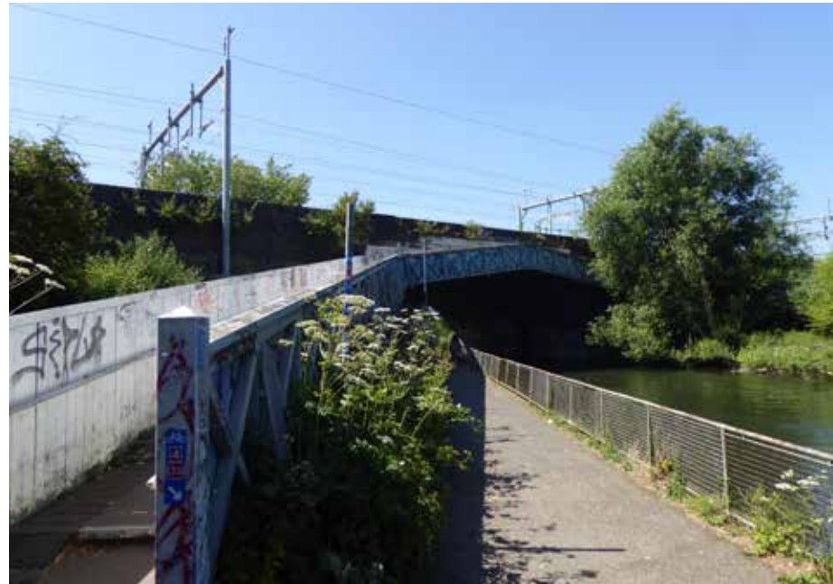
Figure 5.7 View of the Grade II listed railway bridge to the east of the Site.
