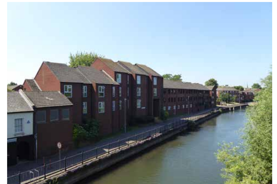
Figure 6.16 Development and river path on the south side of the river opposite the Site.
