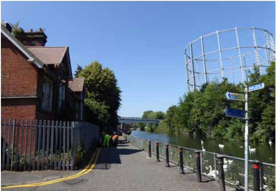
Figure 5.5 The northern boundary of the Grade II listed school plot including river and river pathways. The school is located to the left in this view.
