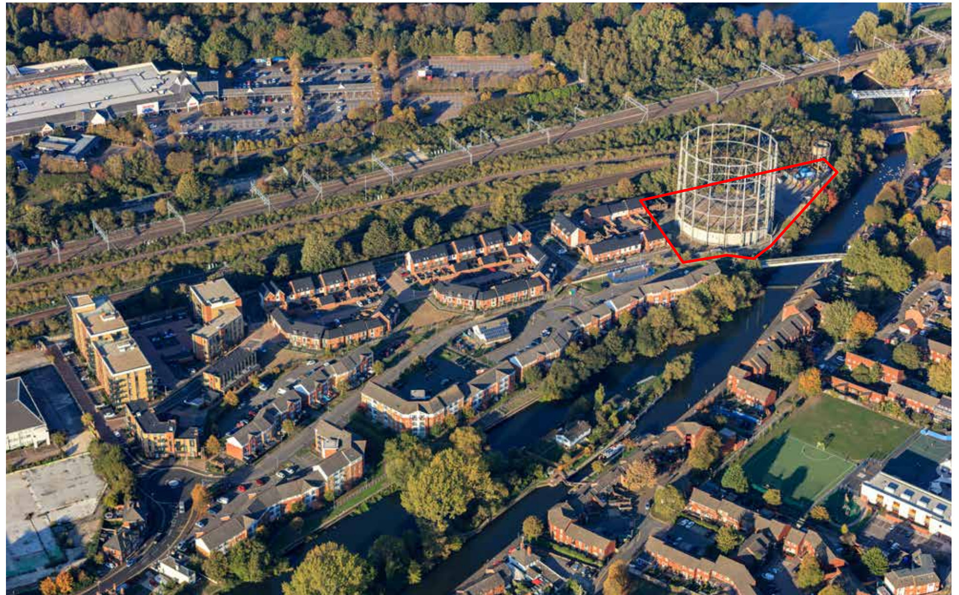
Figure 0.1 Aerial photograph of the Site from the south west showing the existing gasholder
