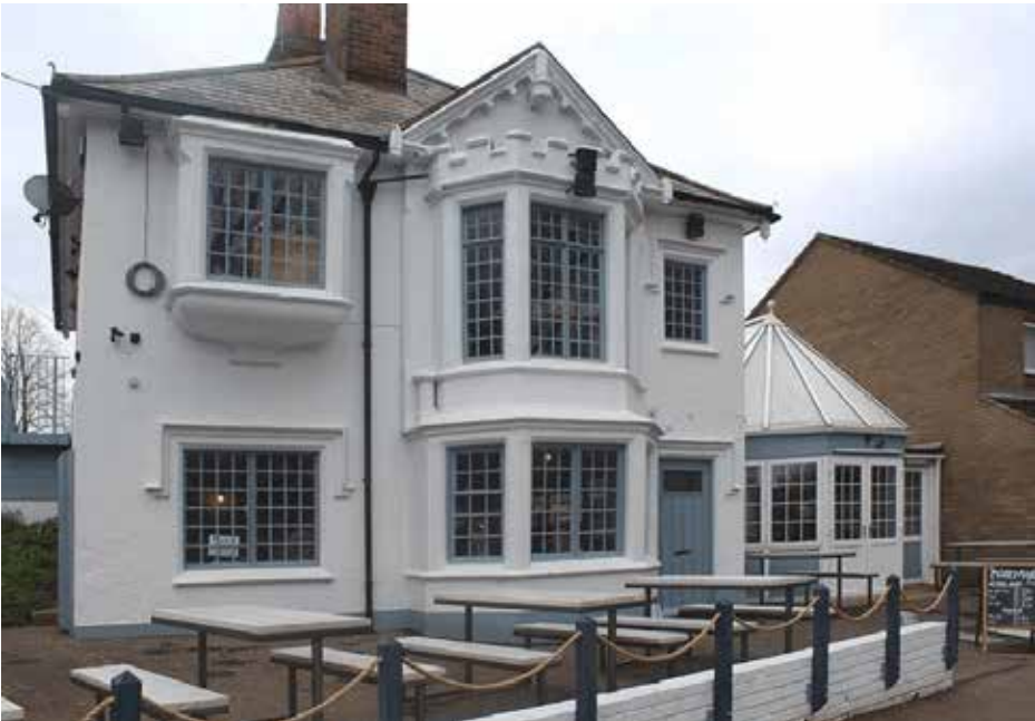
Figure 5.16 North elevation of Fisherman's Cottage Inn (Grade II).
