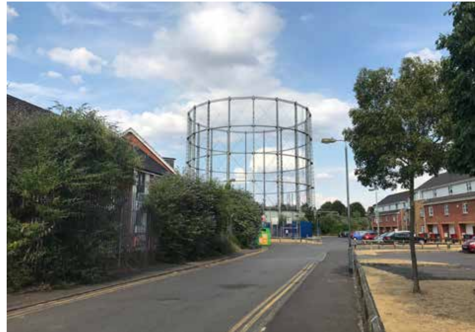
Figure 6.6 The gas holder as seen from within Character Area A.
