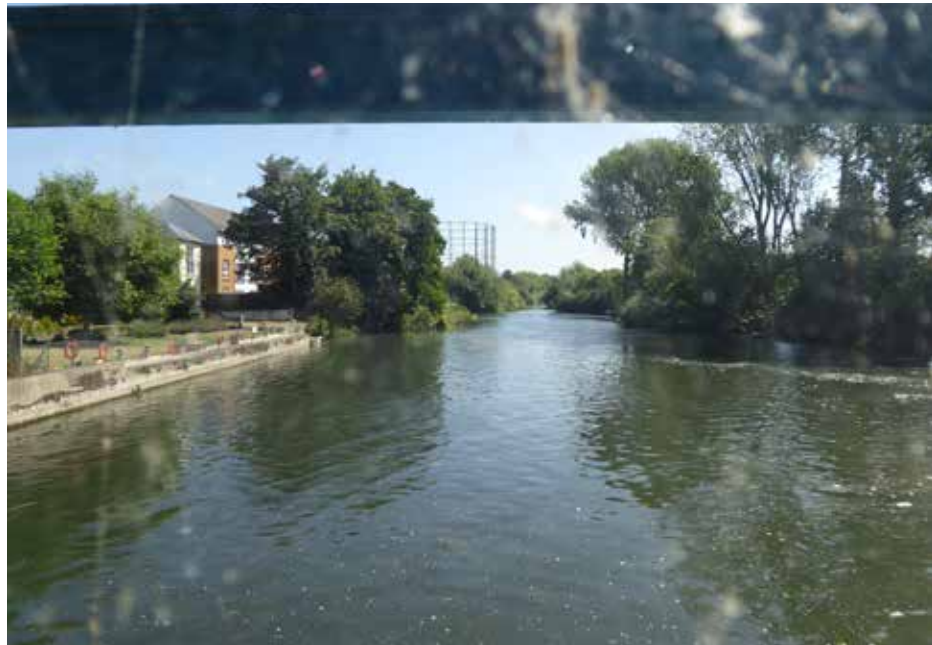
Figure 5.12 The view east along the river from the Pump House and Engine House.
