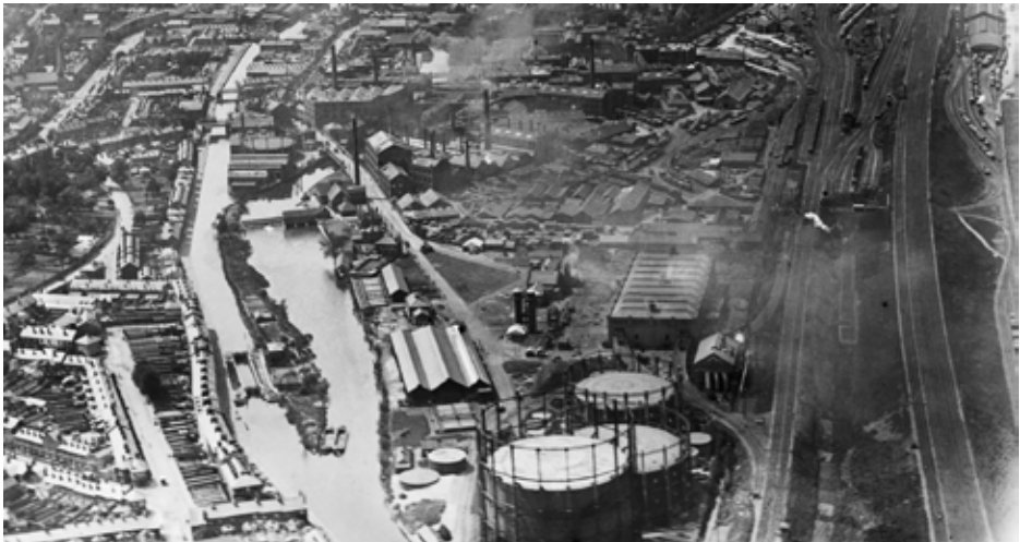
Figure 4.5 Aerial photograph of Reading gasworks from the east, 1920. The remaining gas holder on the Site is identified in red.
