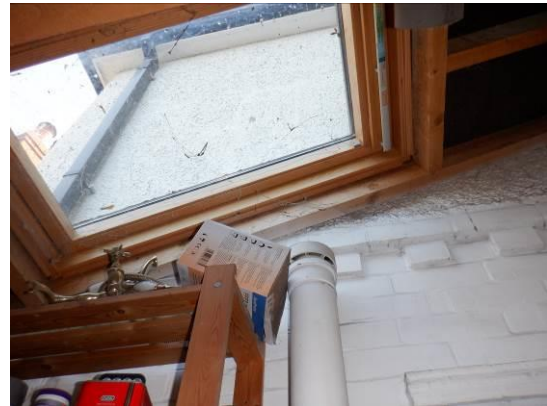
22. Roof light in garage roof.
