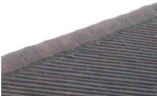
5. Hip tiles securely mortared in place (front elevation).
