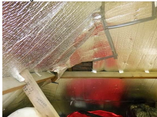
16. Foil bubble wrap insulation tacked to roof rafters.
