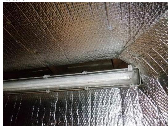
18. Space between ridge tiles and ridge beam.
