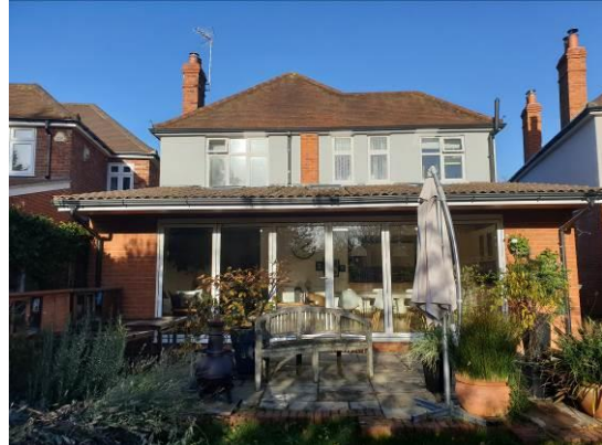
2. Rear of property viewed from southwest.
