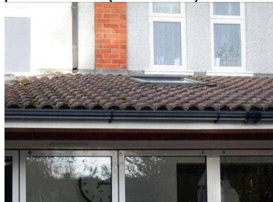
12. Tight interlocking roof tiles on rear extension (rear elevation).
