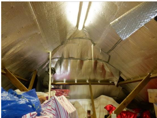
15. Roof void viewed from rear hipped end.
