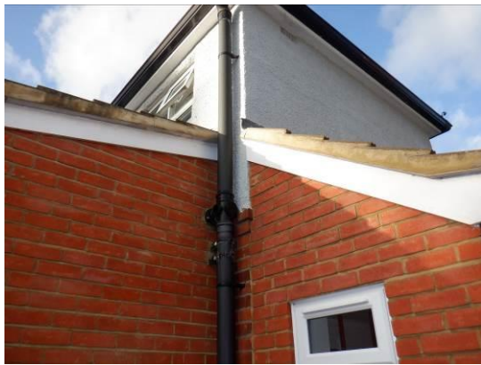
13. Rear and side extensions with intact verge mortar.
