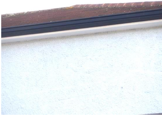
7. Walls rendered up to soffits (southeast elevation).
