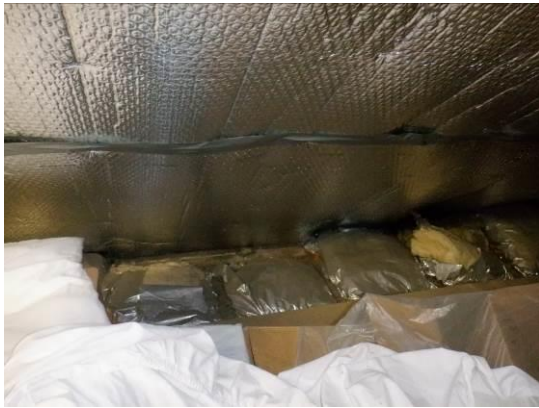
19. Foil wrapped fibreglass at northwest eaves.
