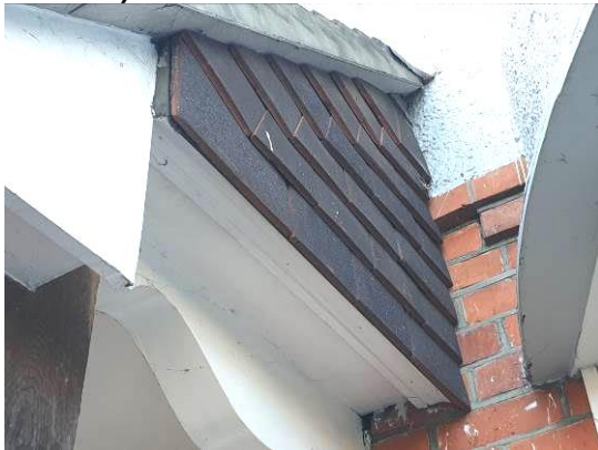
9. Tight hanging tiles on sides of porch roof (northwest elevation).
