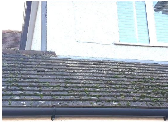
8. Front porch and garage roof (front elevation).
