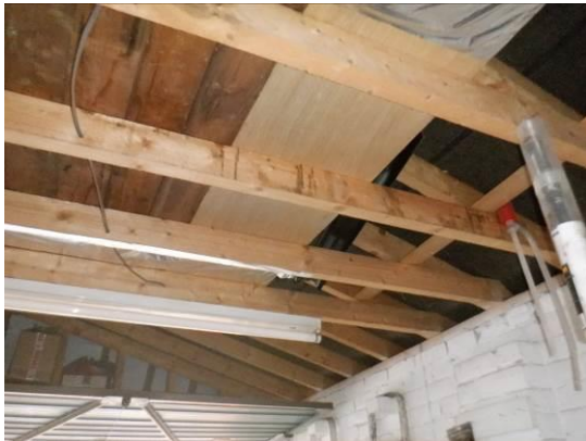
21. Open garage roof.
