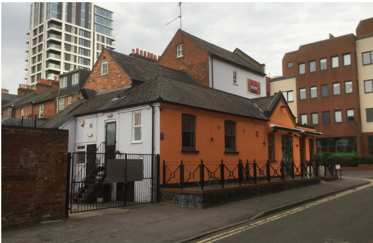
Photograph 2. The northwest facing elevation of the building at 77-79 Kings Road, Reading.
