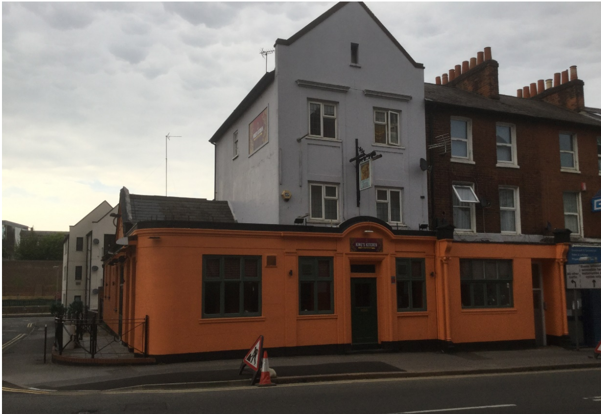
Photograph 1. The south facing elevation of the building at 77-79 Kings Road, Reading.
