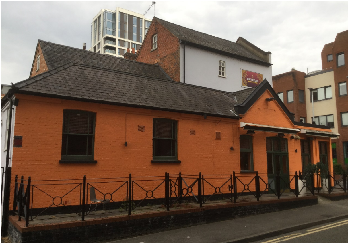
Photograph 3. The west elevation of the building at 77-79 Kings Road, Reading.
