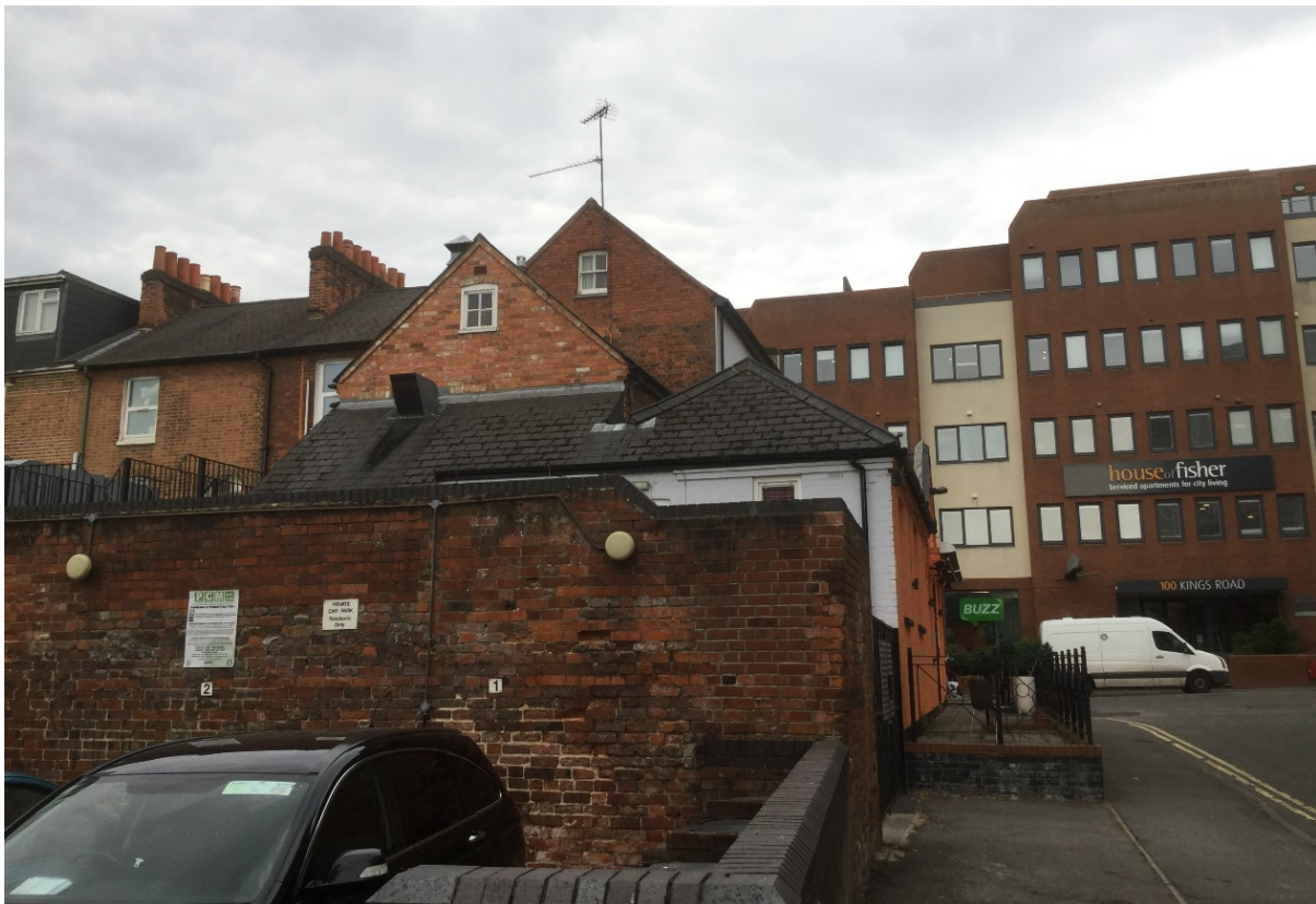
Photograph 4. The south facing elevation of the building at 77-79 Kings Road, Reading.
