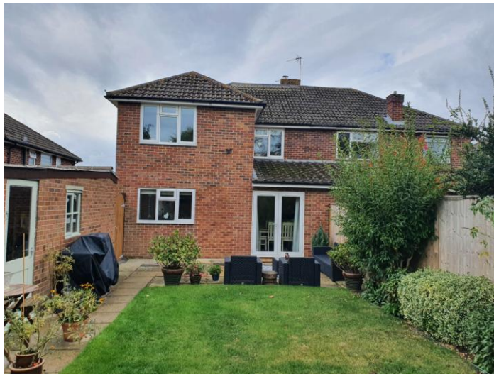
Rear of 49 Elmstone Drive
