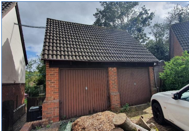
1. Front of garage/outbuilding. Photo provided by the agent on 07/10/2020.
