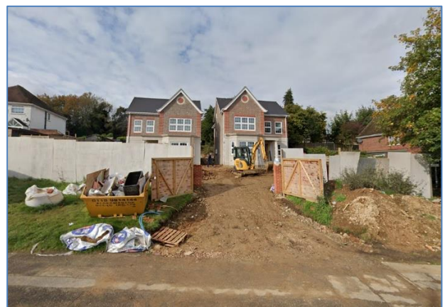
6. Construction in progress at 181 Kentwood Hill. Image captured in October 2020, retrieved from Google Maps on 14/01/2021.
