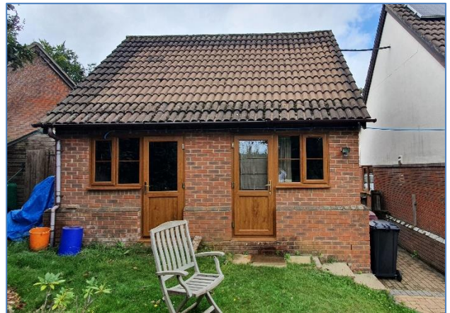
2. Rear of garage/outbuilding. Photo provided by the agent on 07/10/2020.
