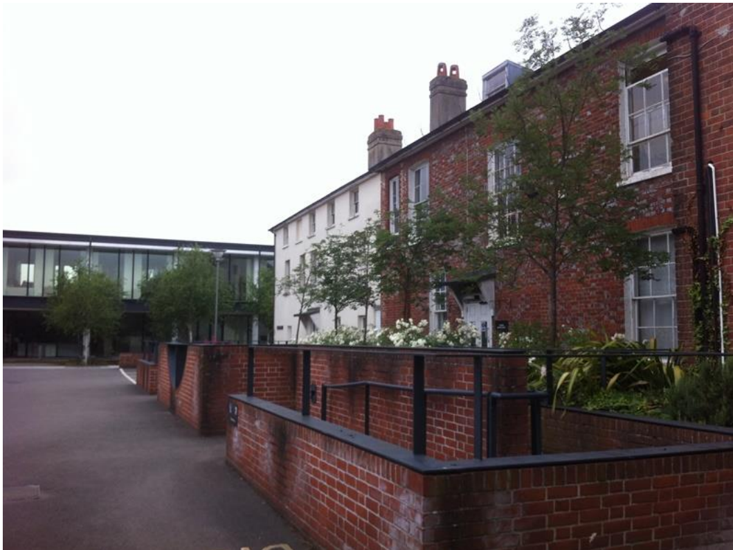
Figure 8: Rear, north elevation, adjacent contemporary Records Office building
