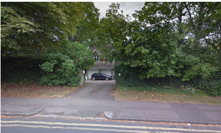
Figure 1 – street view of entrance to the site from Parkside Road
