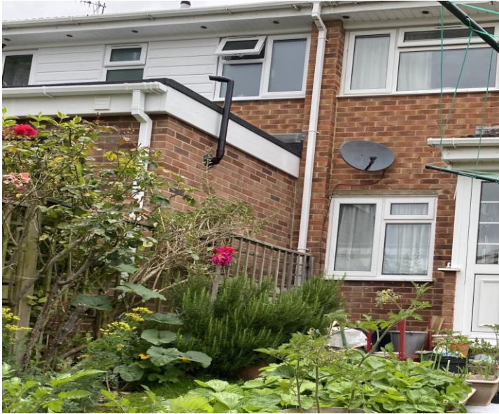
Figure 2: View of the extension from the neighbour's garden
