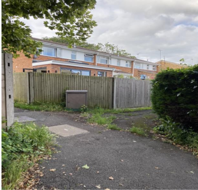
Figure 1: View of the extension from a footpath
