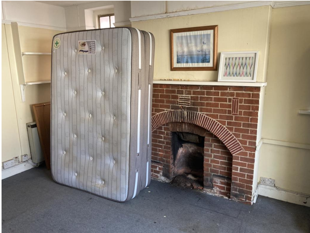
Plate 7: View of fireplace, interior of Bungalow (front building).
