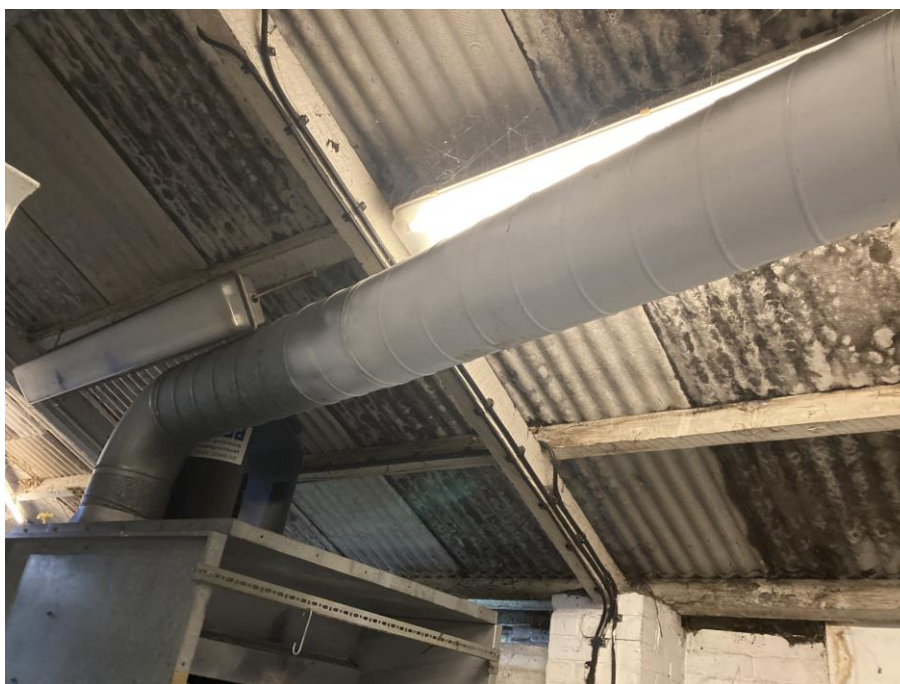
Plate 12: View of extractor pipework and corrugated roof within industrial (rear) building.
