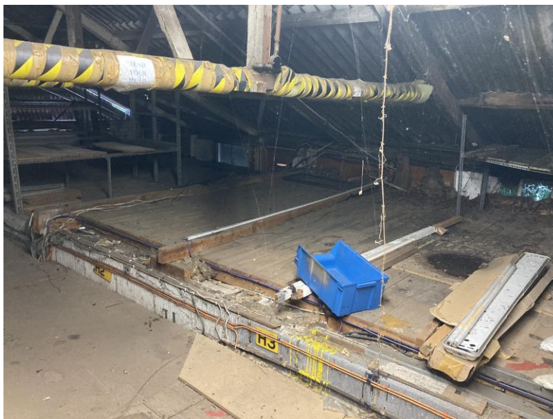
Plate 10: View of mezzanine with corrugated roof above industrial (rear) building.
