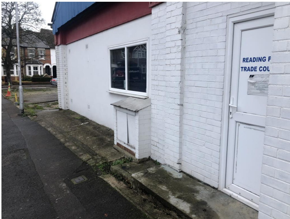
Plate 6: View of west side of site building adjoining Send Road, view facing north-east.
