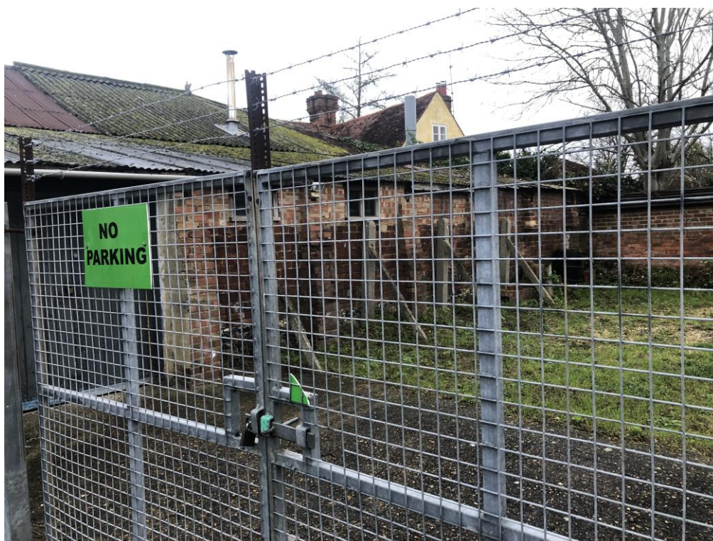
Plate 4: View of site building rear and rear area (gated), view facing north-east.
