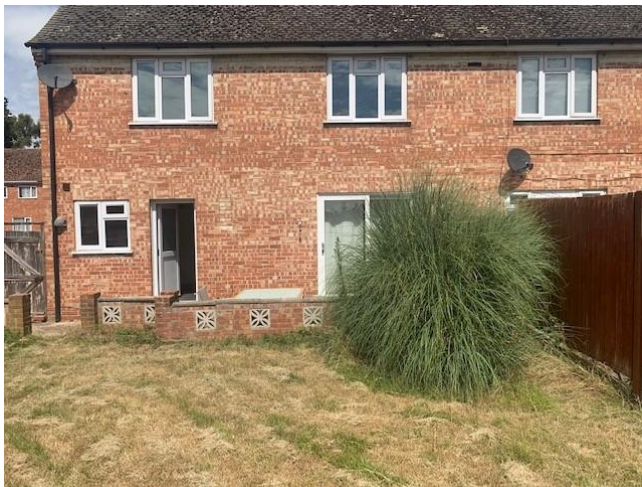
1. Rear elevation of 82 Ambrook Road (image supplied by applicant).
