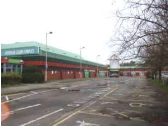
1. Front of Rivermead Leisure Centre viewed from southeast.
