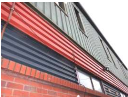
7. Tightly bolted metal cladding (western elevation).
