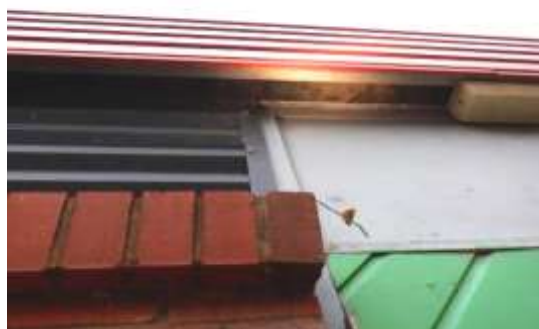
12. Mesh and fibreglass under pool roof overhang (eastern elevation).
