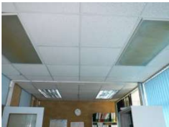
19. False ceiling tiles in office.
