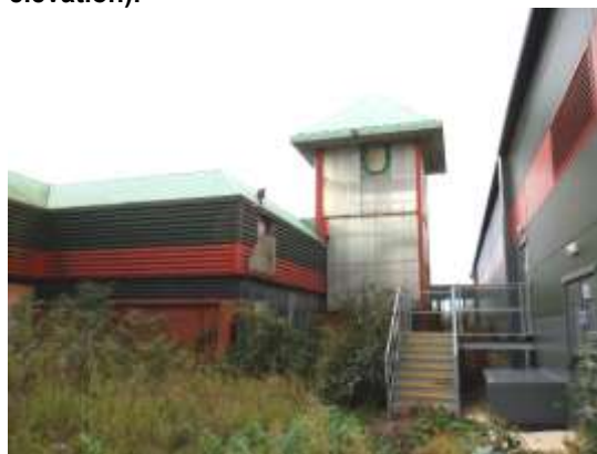
10. Water slide removed from tower (eastern elevation).
