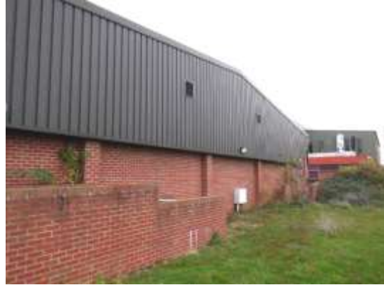
2. Brick walls with metal cladding above on the gym (western elevation).
