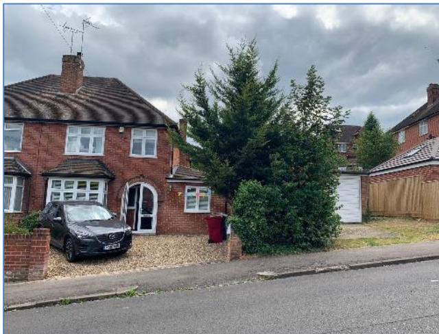
1. Existing front elevation - 43 Oakley Road
