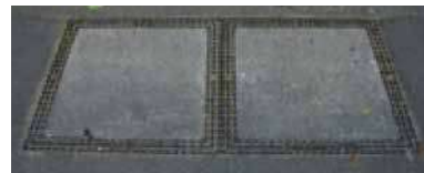
JF6 old cast and concrete type 70x140cm
