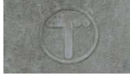
Fibreglass Telecom marking
