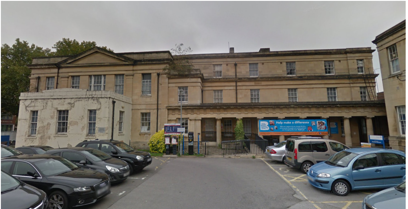
Figure 4 - Old Maids Building Western Face - Captured October 2018 (Source: Google Street View)
