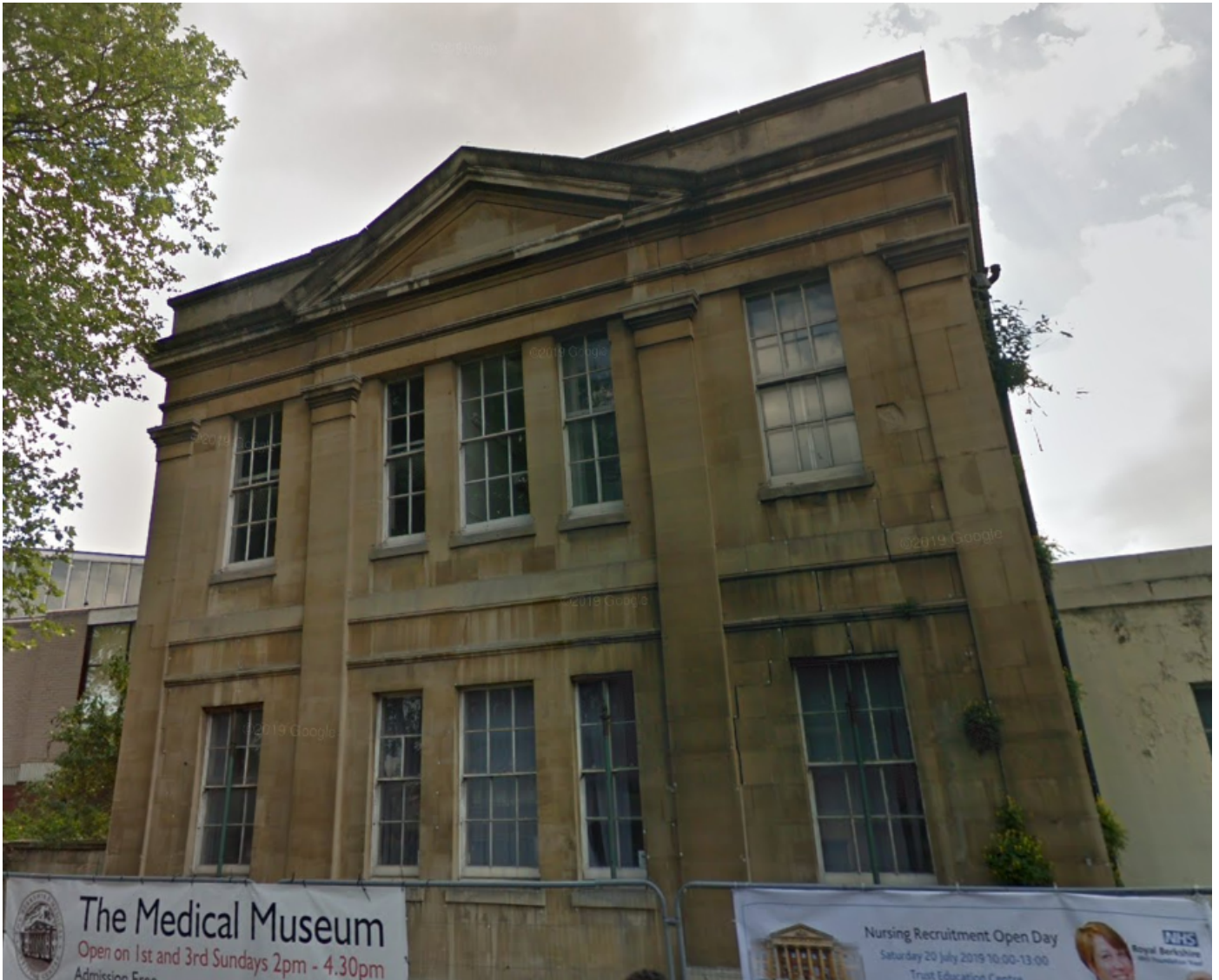
Figure 3 - Old Maids Building Northern Face – Captured May 2019 (Source: Google Street View)
