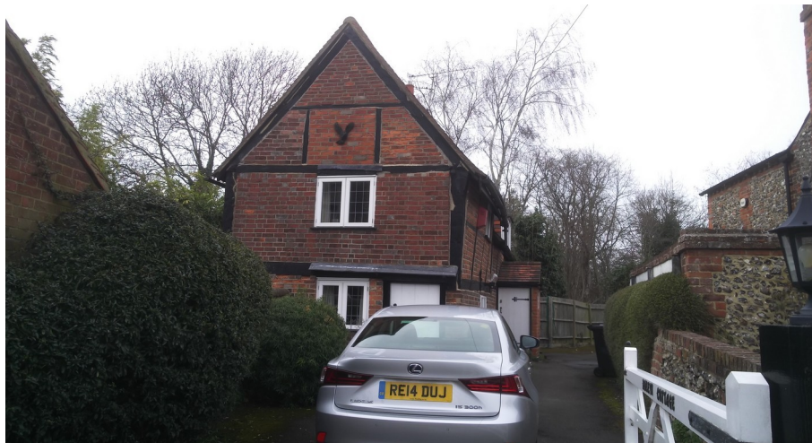
Picture 1 – House Frontage to Paddock Road.
