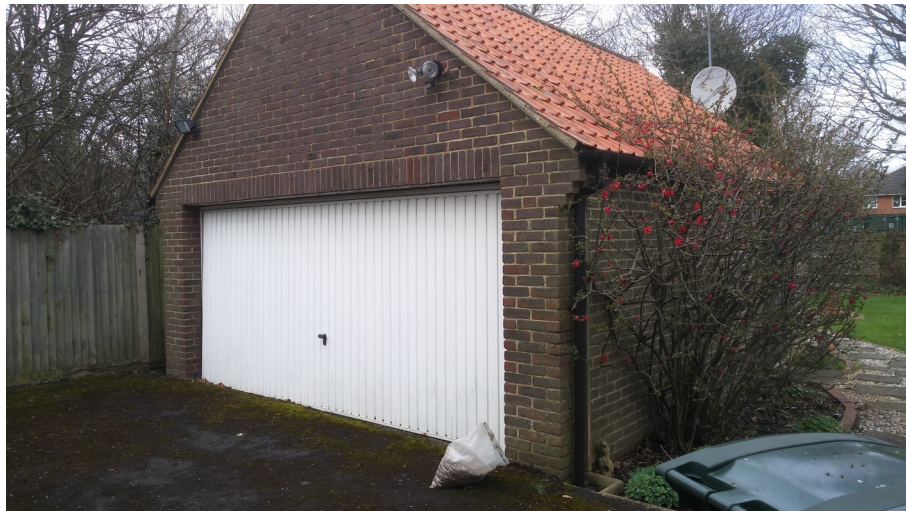
Picture 2 – Detached garage.
