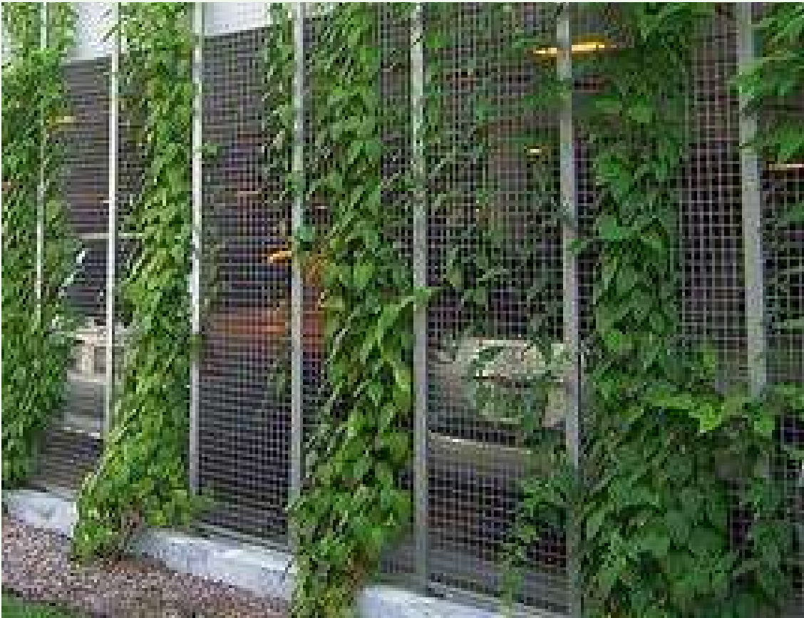
PRECEDENT IMAGES OF THE CABLE TRELLIS
